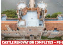
CASTLE RENOVATION COMPLETES – P8-9
