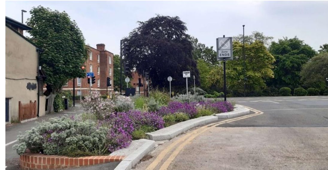
Figure 83: Raingarden introduced into the street which incorporates wildflowers and helps manage surface water run-off
