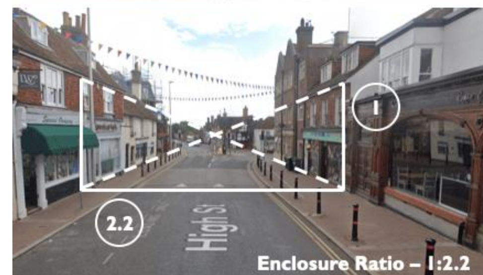
Figure 40: Enclosure ratio of different sections of the High Street. This is typically in the order of 1:2 along much of the High Street, though extending significantly in the vicinity of Vicarage Fields (image source: Google Streetview image capture © 2024)
