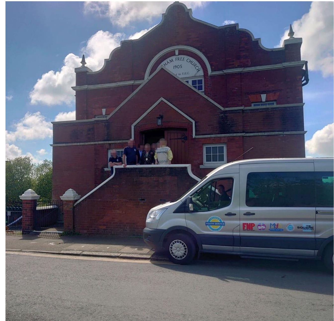
Figure 26: The former Hailsham Free Church building is a good local example of a building being repurposed and given new life following adaptation as the Station Youth Centre.
