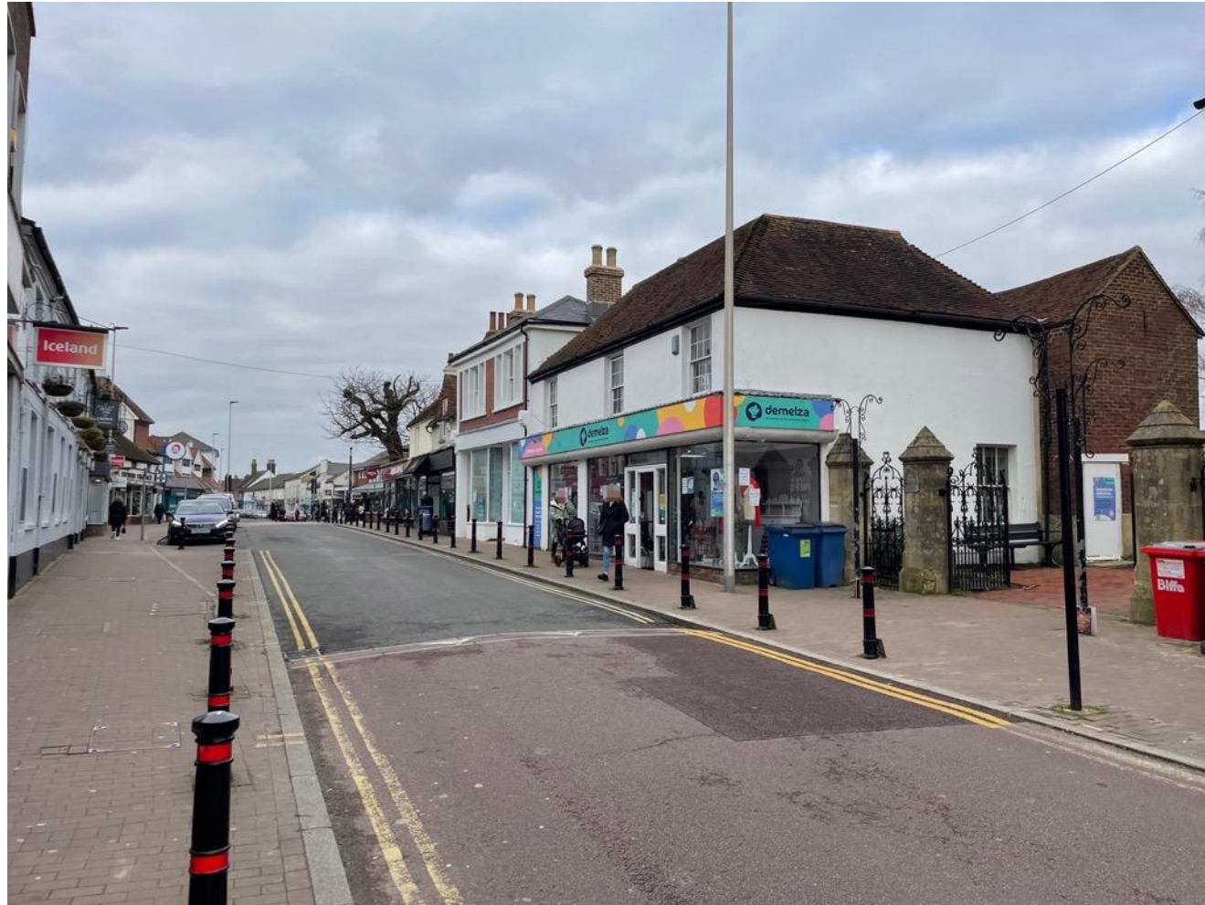
Figure 28: View looking north along Hailsham High Street
