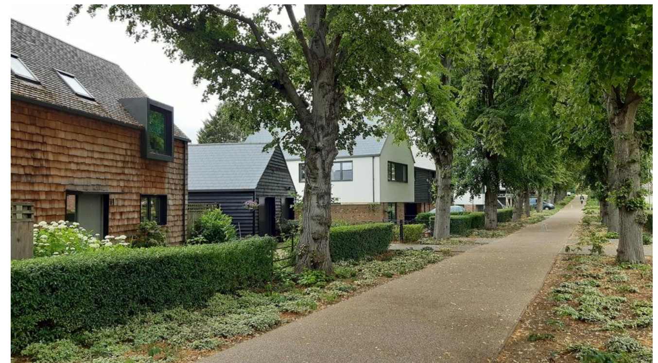
Figure 54: The Avenue, in Saffron Walden, is a good example of a development that uses a limited palette of locally distinctive materials and colours in a variety of ways and combinations to create interest and character. Retention of mature trees and use of soft landscaping with the street environment and along property boundaries further enriches the quality of development.
