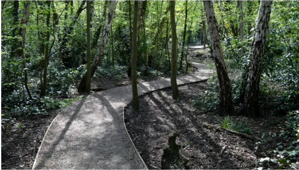
Figure 4: An example of a bound gravel 'no dig' path through a woodland. NB: this example does not include the edge fencing proposed in the appeal scheme.
