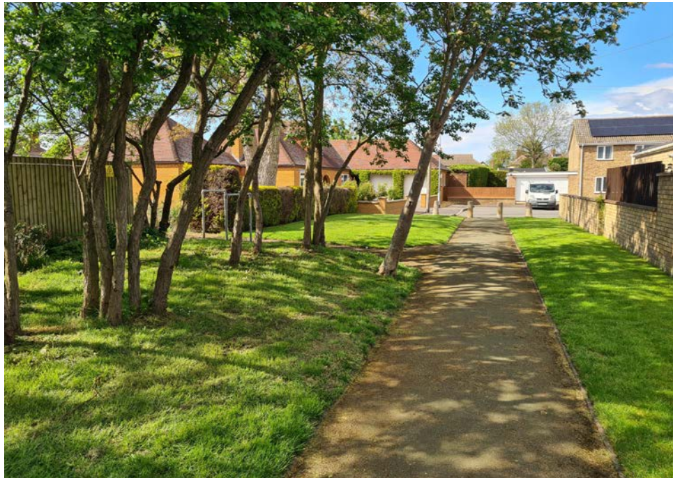
FUNCTIONAL SOUTHERN PRoW IN TAR SPRAY AND CHIP THROUGH GENEROUS LANDSCAPED CORRIDOR
