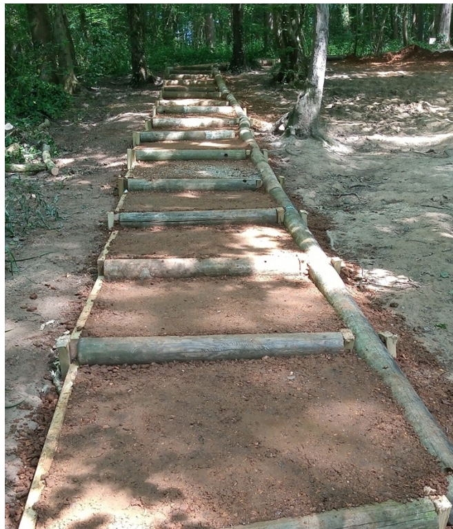
Figure 5: An example of a bound gravel path on a slope through a woodland and held in place with timber. NB: this example does not include the edge fencing proposed as part of the appeal scheme.
