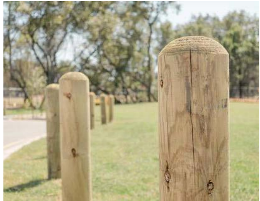
LOW TIMBER BOLLARDS ALONG GREEN VERGE TO PREVENT VEHICULAR OVERRUN
