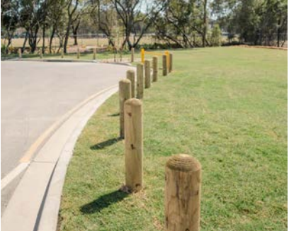
BOLLARDS PROTECTING POS VERGE
