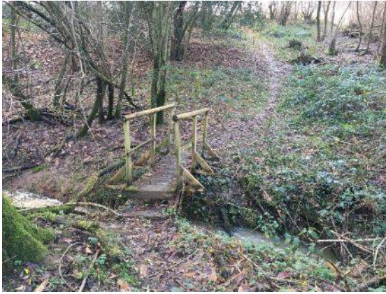
Photograph 7. Existing footbridge over stream, along footpath through ASNW W2.
