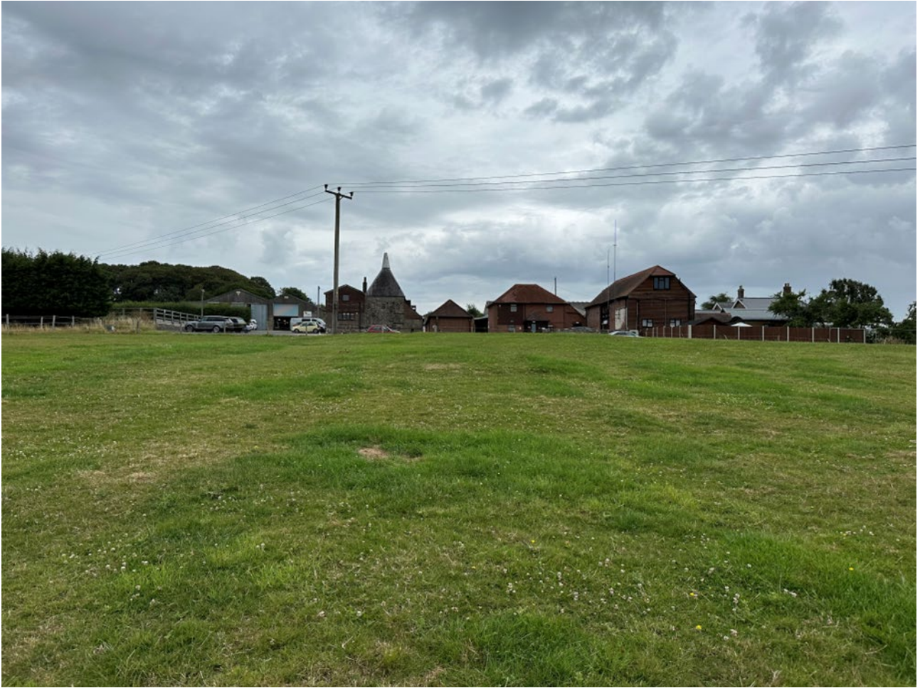
Plate 1: The Oast House and neighbouring farm buildings seen from within the area of the Appeal Site to the west. The original form of the listed building is visible, with the square stone building topped with a steeply pitched roof and cowl above. The timber clad, 20 th century cooling room is visible to the left (north). The former farmhouse and historic barn are visible to the right (south). This area of the Site will be retained as open space, with this view retained and made publicly accessible. The understanding of the Oast House may be aided by interpretation boards and information.
