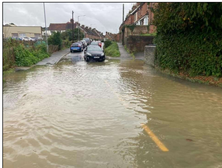
Figure 6.2: Flooding on Framfield Road (looking west near Community Hospital)
