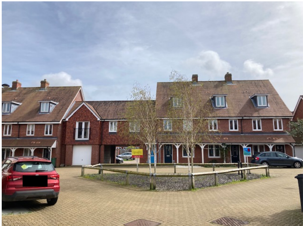
Terrace of town houses and apartments at Hawksley Crescent, Welbury Meadows
