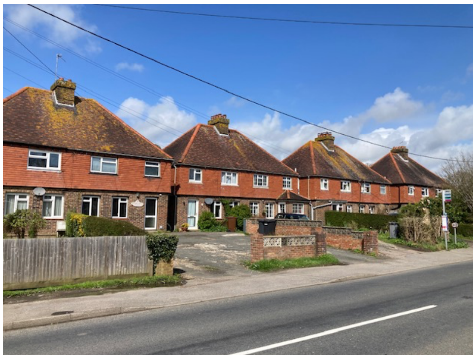
Brookland Terrace on the northern side of the A271, Lower Horsebridge.
