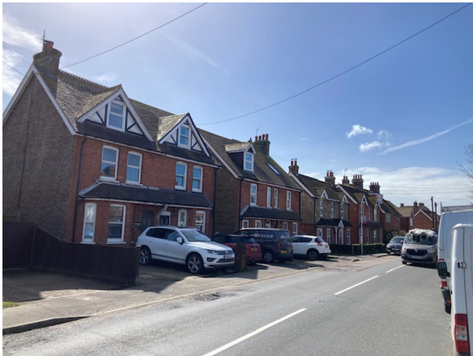
Houses on the southern side of the A271, Lower Horsebridge. These are identified as 'positive buildings' on Map 4 of the HNP (CD 5.4 page 65).
