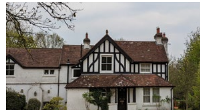
Timber frame and white render infills
