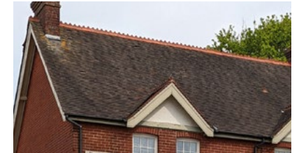
Gabled roof with dark slates
