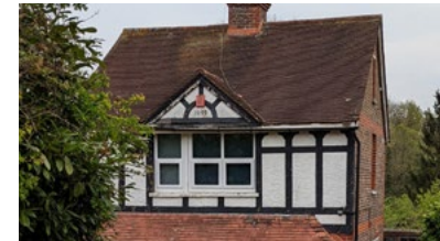
Timber frame with white render infills
