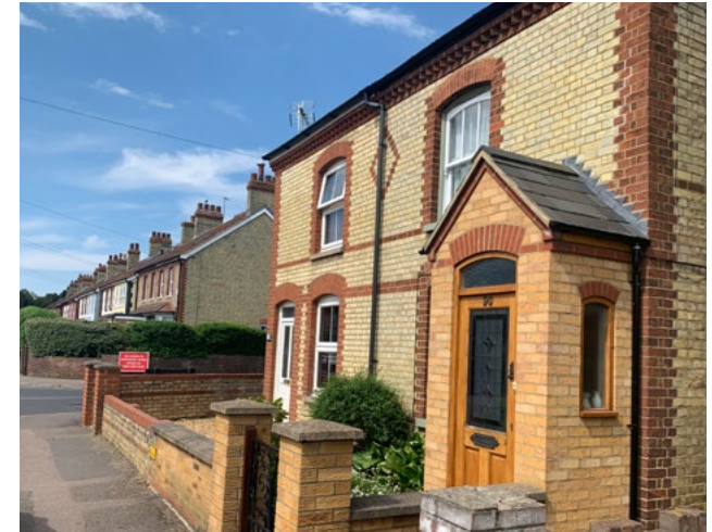
Figure 116: Positive example of a front extension.
