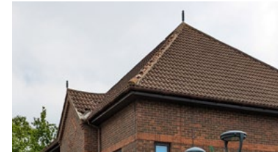
Hipped roof with concrete tiles
