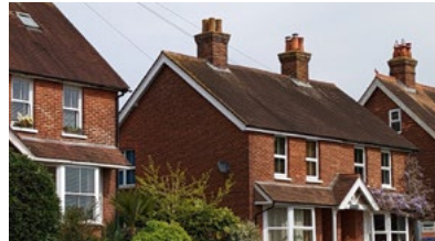
Gabled roof with red clay tiles
