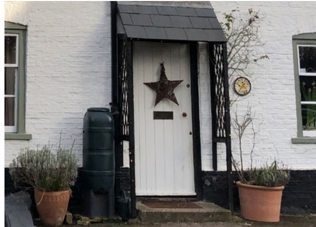
Figure 87: Examples of water butts used for rainwater harvesting in Reach, Cambridgeshire.
