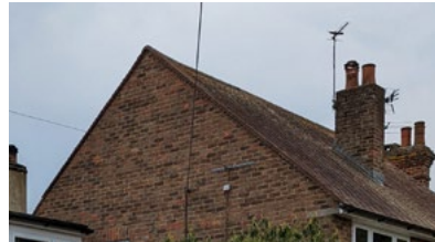
Gabled roof with brown clay tiles
