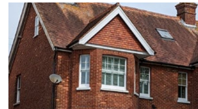
Sash windows with wooden detailing
