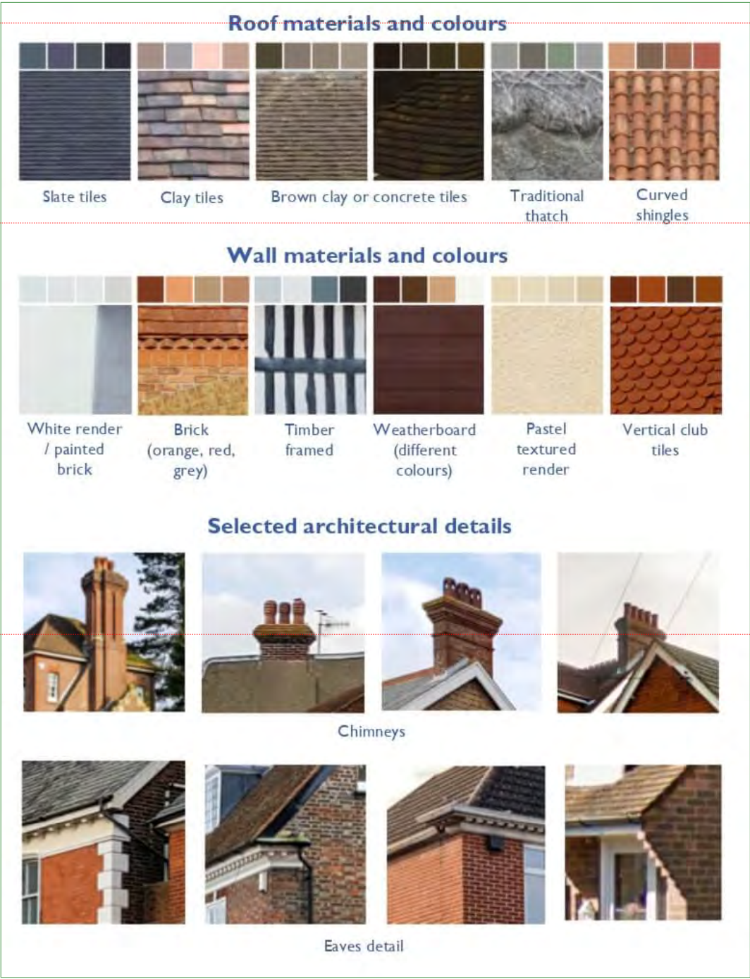
Figure 13: Building materials, colours and details common in Hailsham
