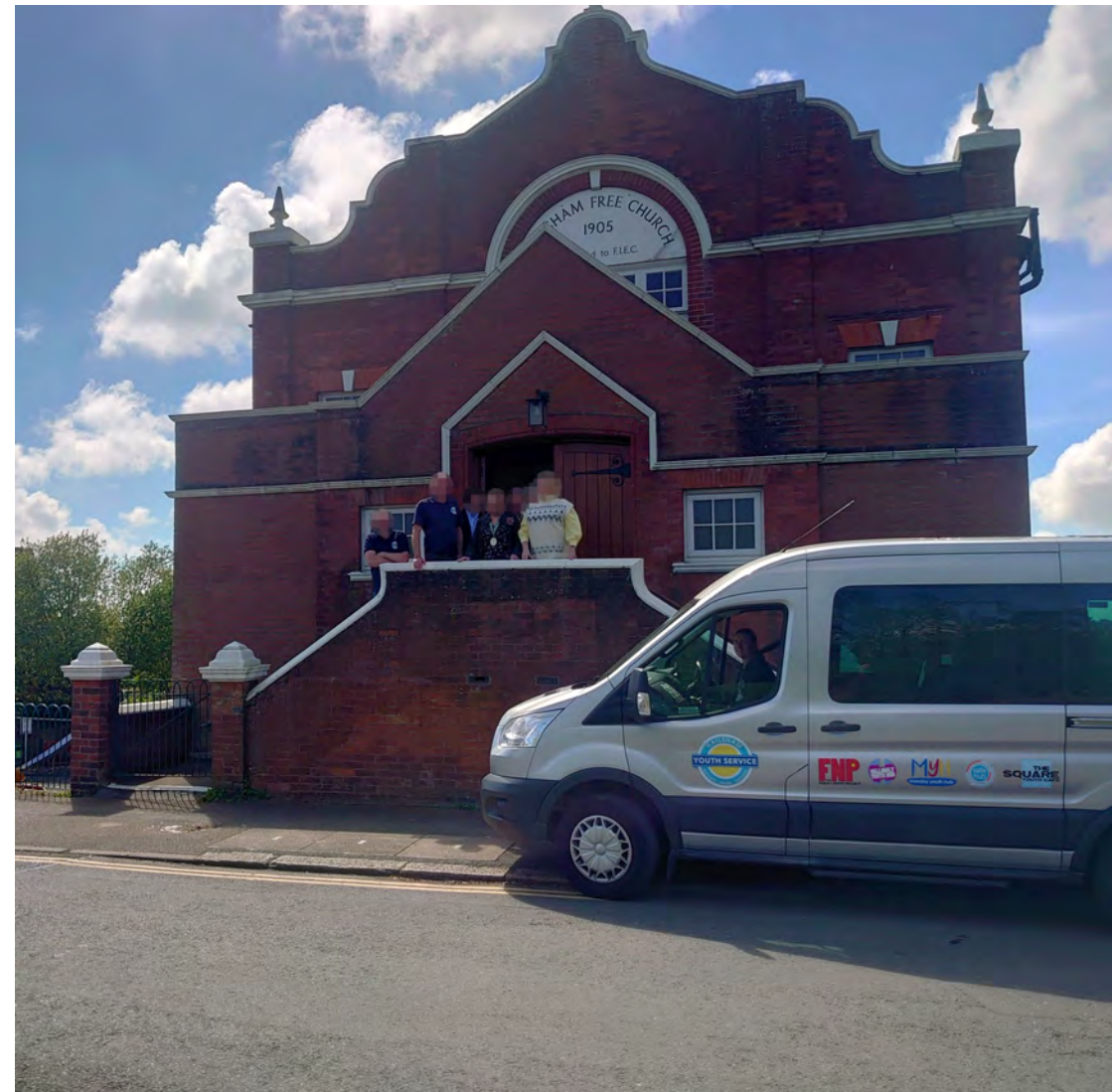
Figure 26: The former Hailsham Free Church building is a good local example of a building being repurposed and given new life following adaptation as the Station Youth Centre.
