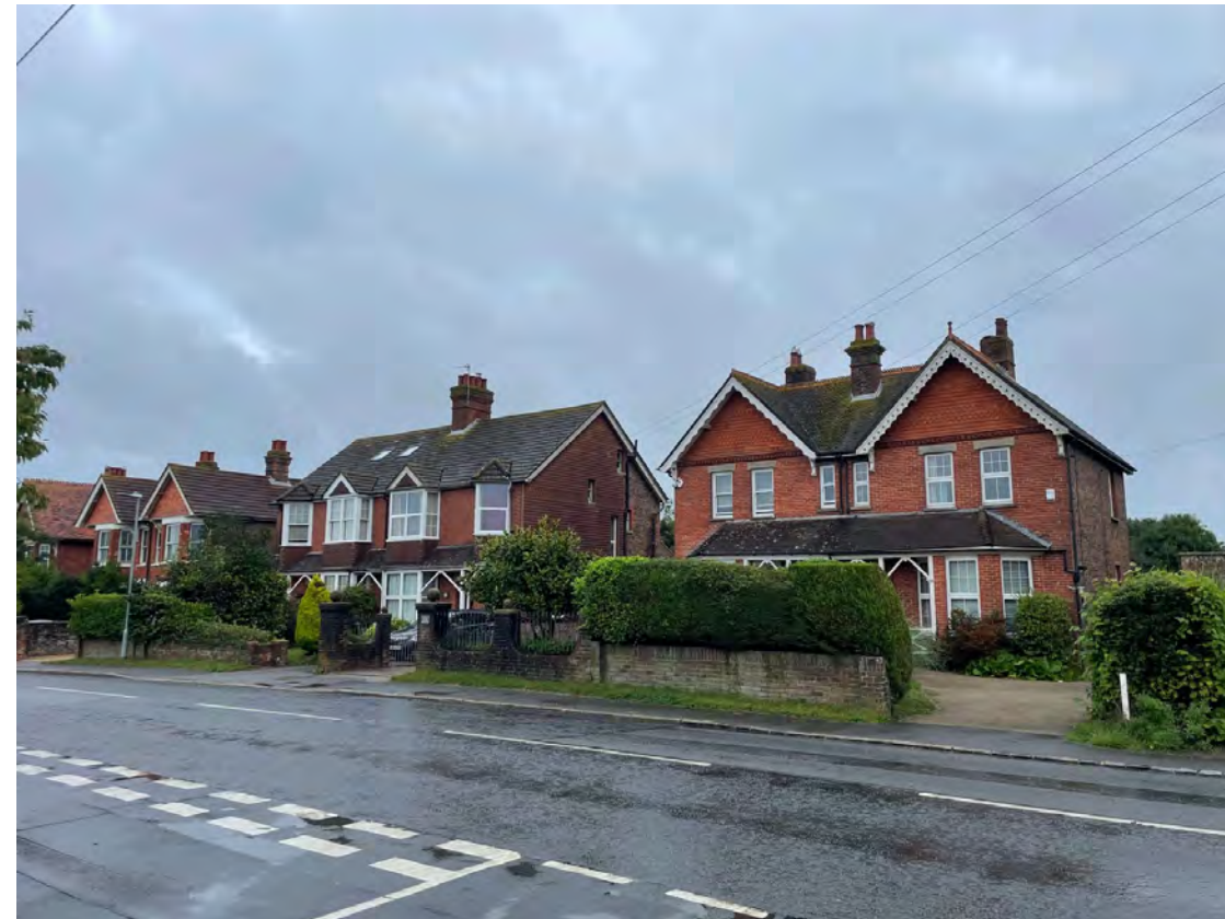
Figure 4.1: Older, more established areas of housing are well integrated within the overall form of development, with street networks creating a permeable structure that supports walking and cycling
