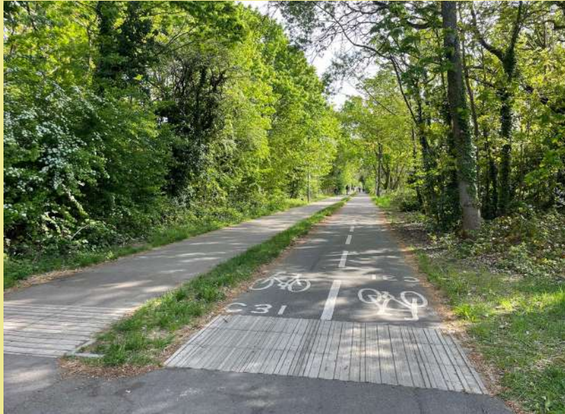
Figure 17: Example of segregated off-road footway and cycleway
