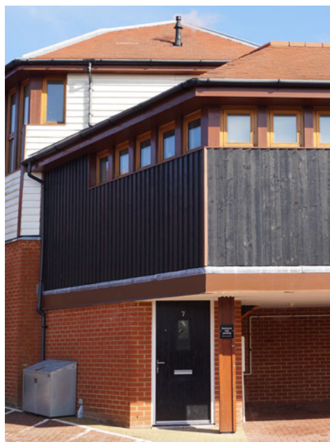
An example of full height weatherboarding (l). Vertical weatherboarding (r) must not be used.
