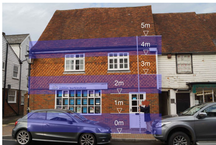
Typical building heights on the High Street.
