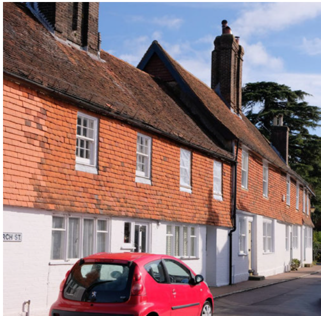
Houses in Church Street with distinctive tiles and steep roofs.
