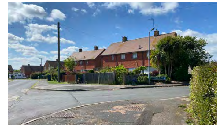
Photo 16: Gabled roofs visible along Park Croft
