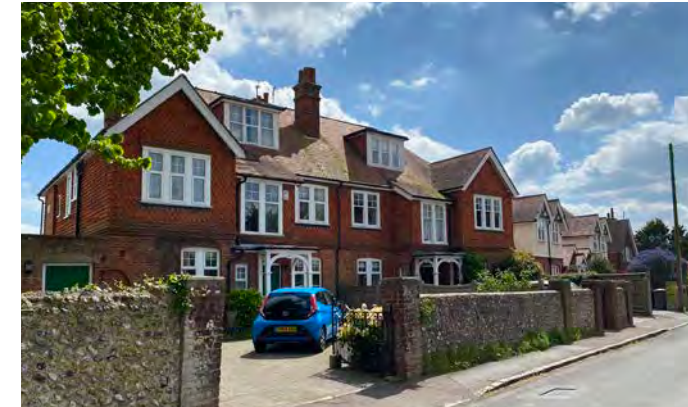
Photo 21: Use of red brick and hanging tiles along Church Street
