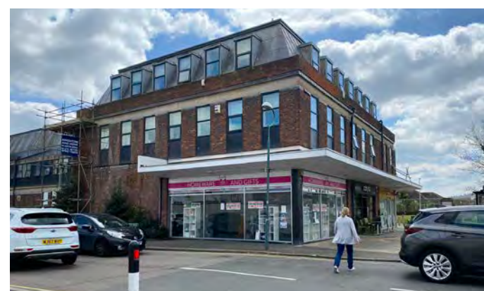
Photo 17: Example of mansard roof along Polegate High Street
