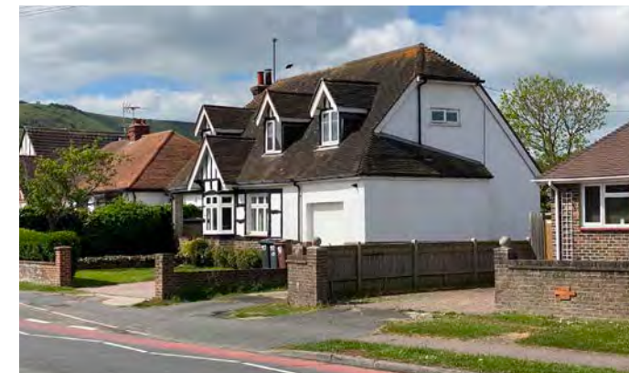
Photo 15: Example of detached housetype with dormer roof
