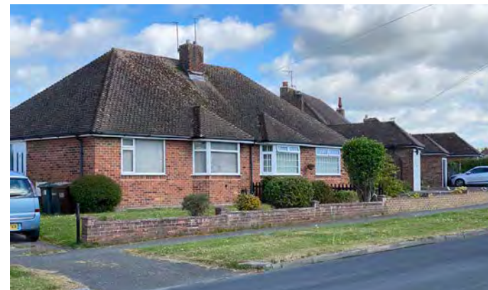
Photo 14: Example of bungalow housetype along Brightling Road
