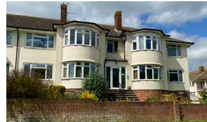
Photo 24: Use of rendering on buildings along Eastbourne Road
