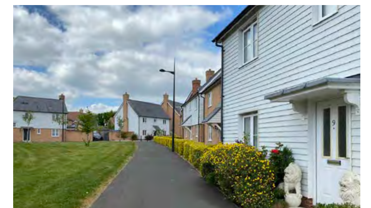
Photo 28: Use of timber weatherboarding within The Mill development
