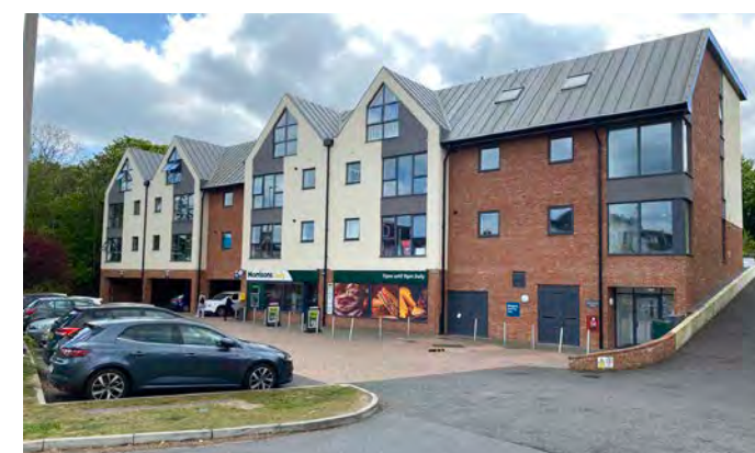
Photo 18: Example of 3-storey apartments above retail along Pevensey Road
