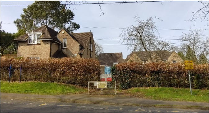
Photo 1: View west from along Scotsford Road with the former school building and school house visible above the foreground hedgerow
