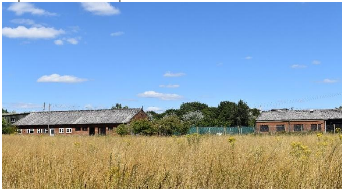
Photo 1: View north from public footpath south of the site, looking towards the existing industrial units along the southern edge of the site
