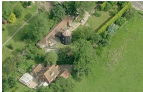
with aerial view
