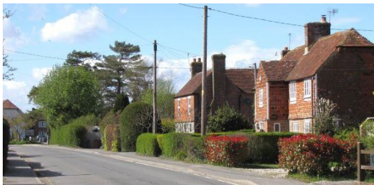
1-3 Fir Tree Cottages & Fir Tree House
