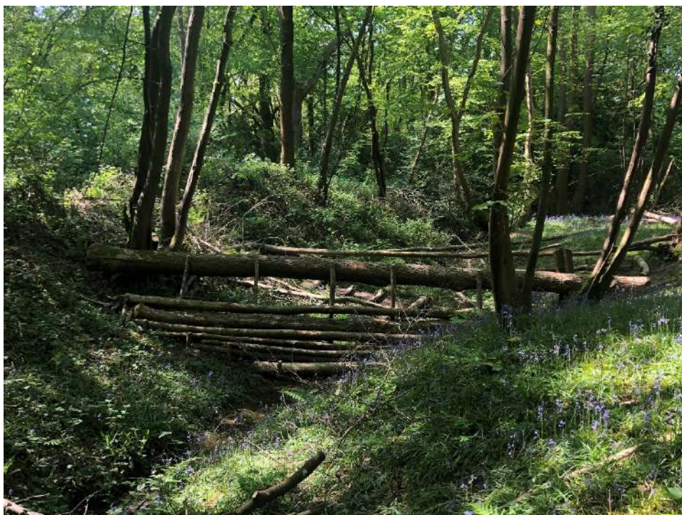
Figure 12 Example of leaky wooden dams recently installed in Sapperton Wood
