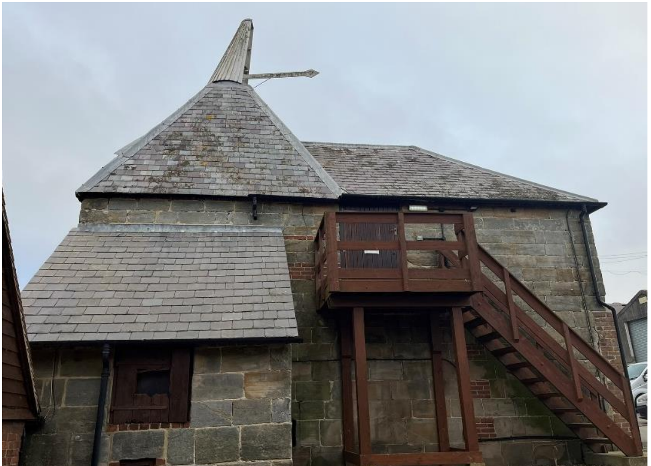
Figure 4.1: Southwest elevation of Oasthouse. Source: Montagu Evans LLP.
