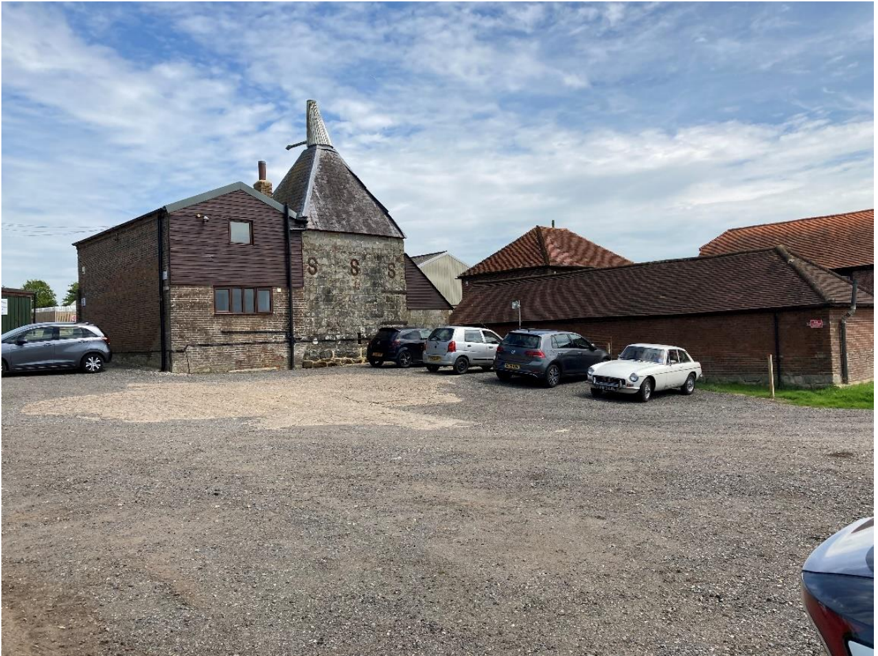
Figure 4.5: Gravel and concrete car park immediately west of oasthouse.
