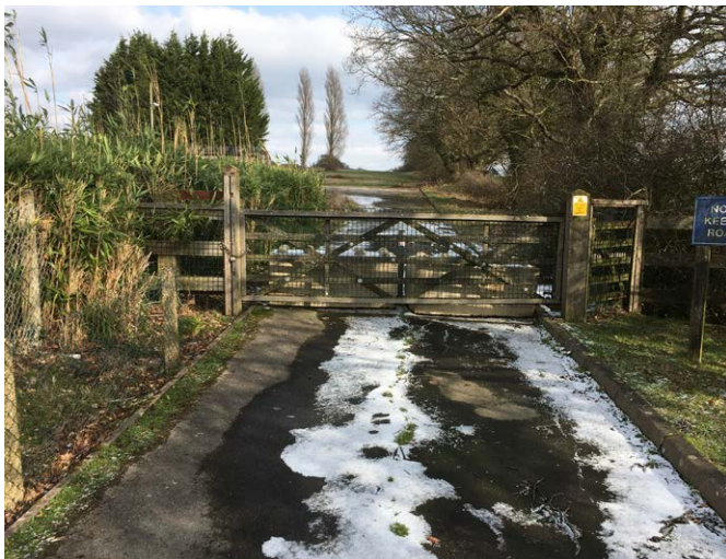
4. Current access to site from Eastbourne Road
