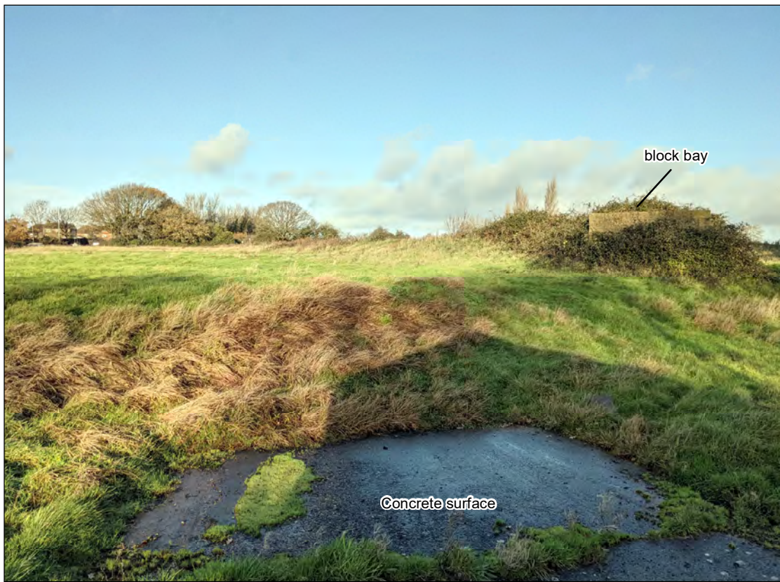
Plate 5) View of the block bay, concrete surface and southern slope of the terrace, facing north
