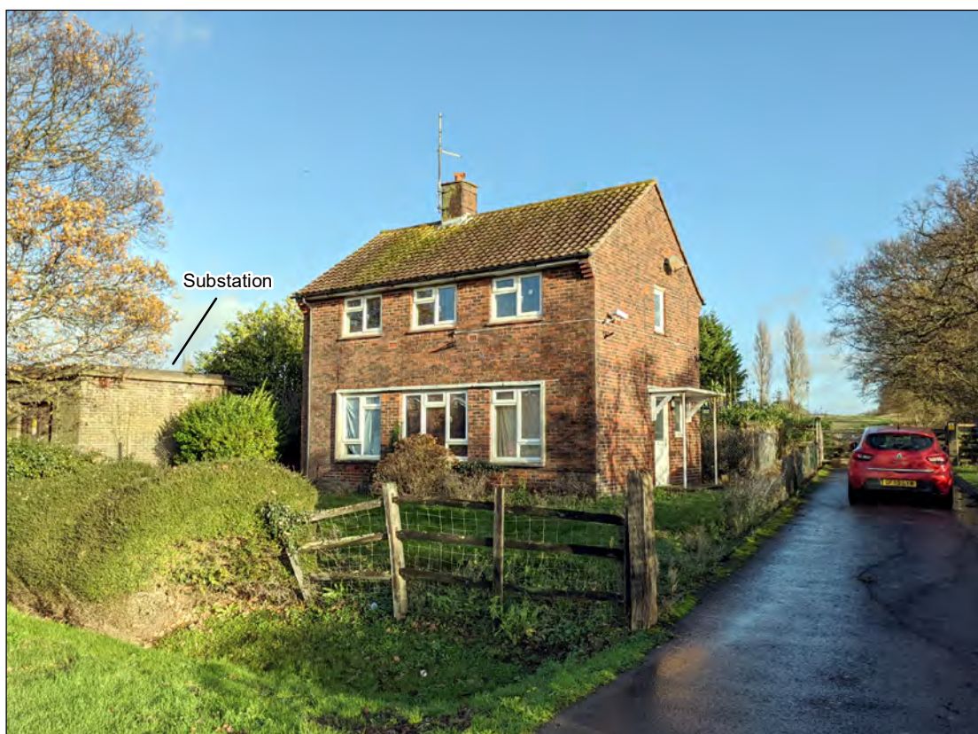
Plate 2) Modern detached house and electric substation located in the southwest corner, facing north
