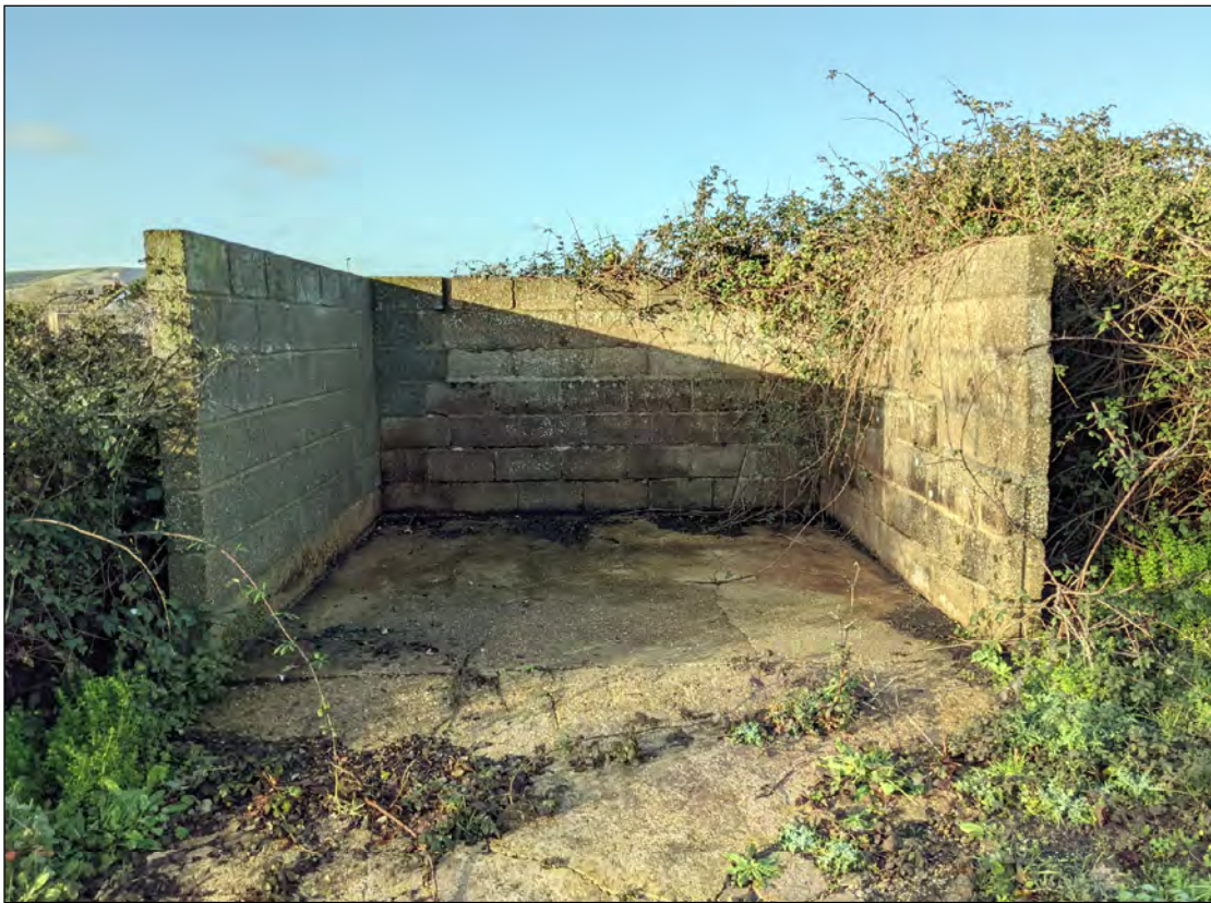
Plate 7) View of the block bay, facing west
