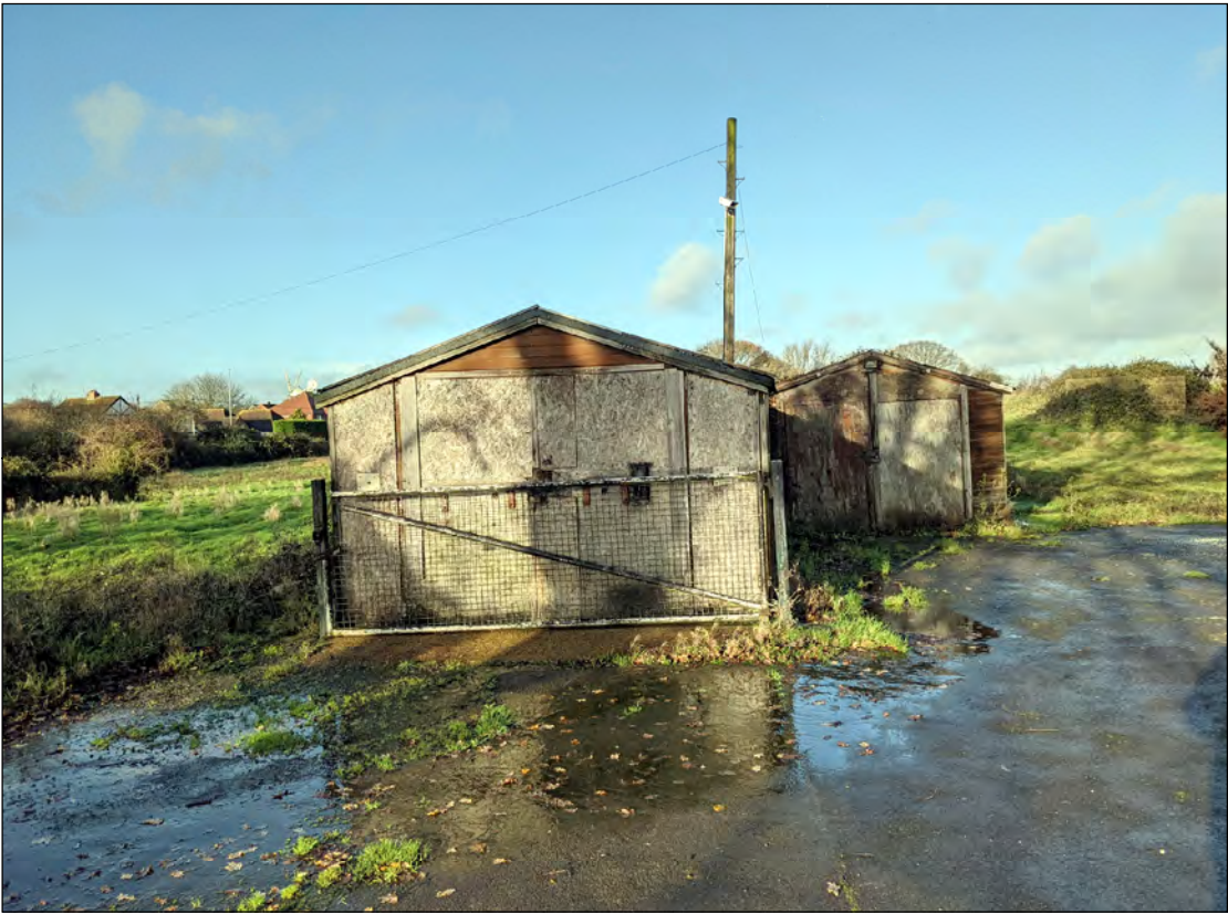
Plate 4) Modern sheds located in the southwest section of the Site, facing west
