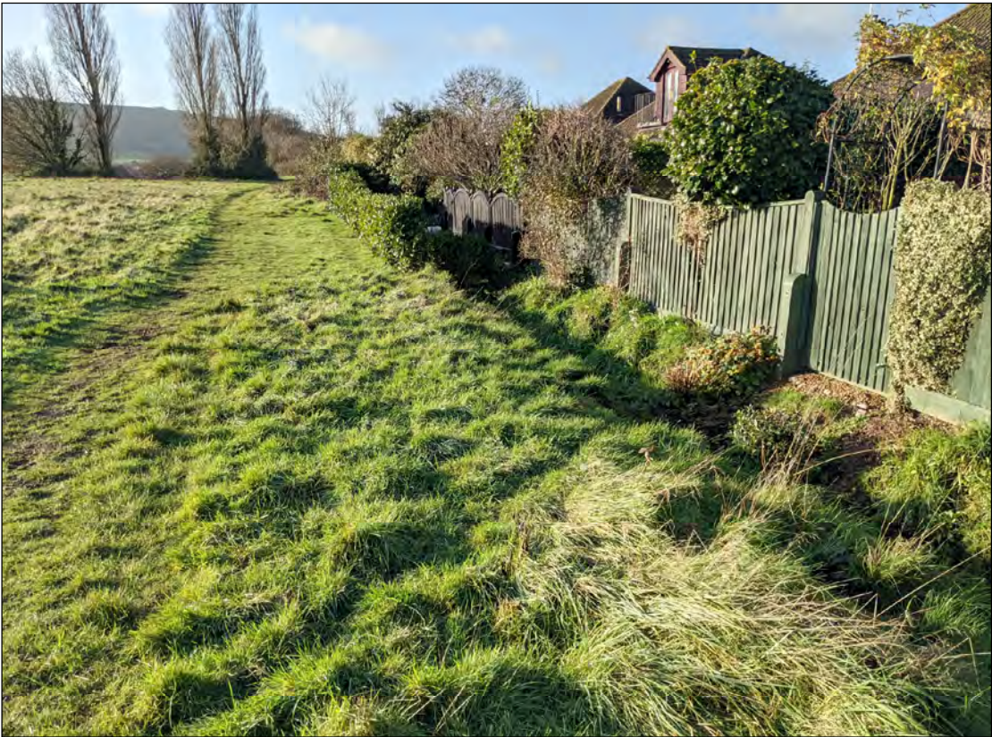
Plate 14) View of the shallow drainage ditch located on the western boundary of the Site, facing southwest
