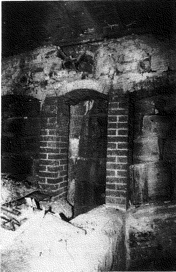
10ii: The north wall of the kiln. The separation of the flues is visible at the lower level. The point at which they entered the chimney is shown at the top: the curved bricks are intact on the east side but have collapsed on the west side.
