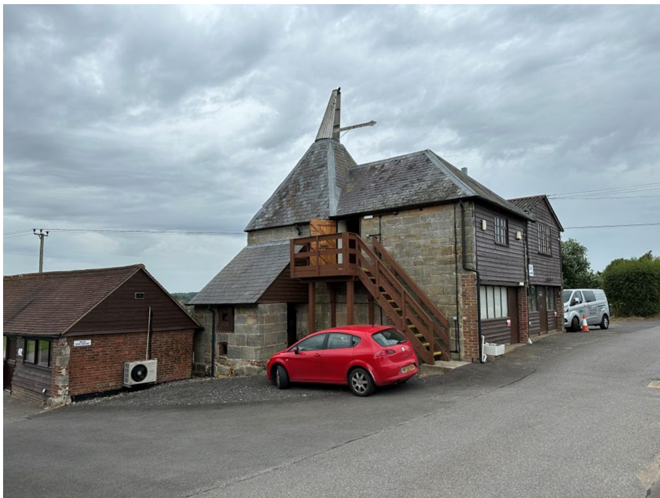
Plate 2: The Oast House viewed from within the farmstead looking north-west. This includes the altered east elevation and the later cooling room to the north.
