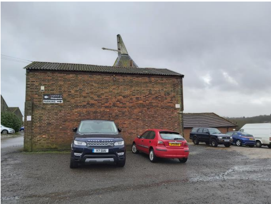
Figure 19: North elevation of The Oast
