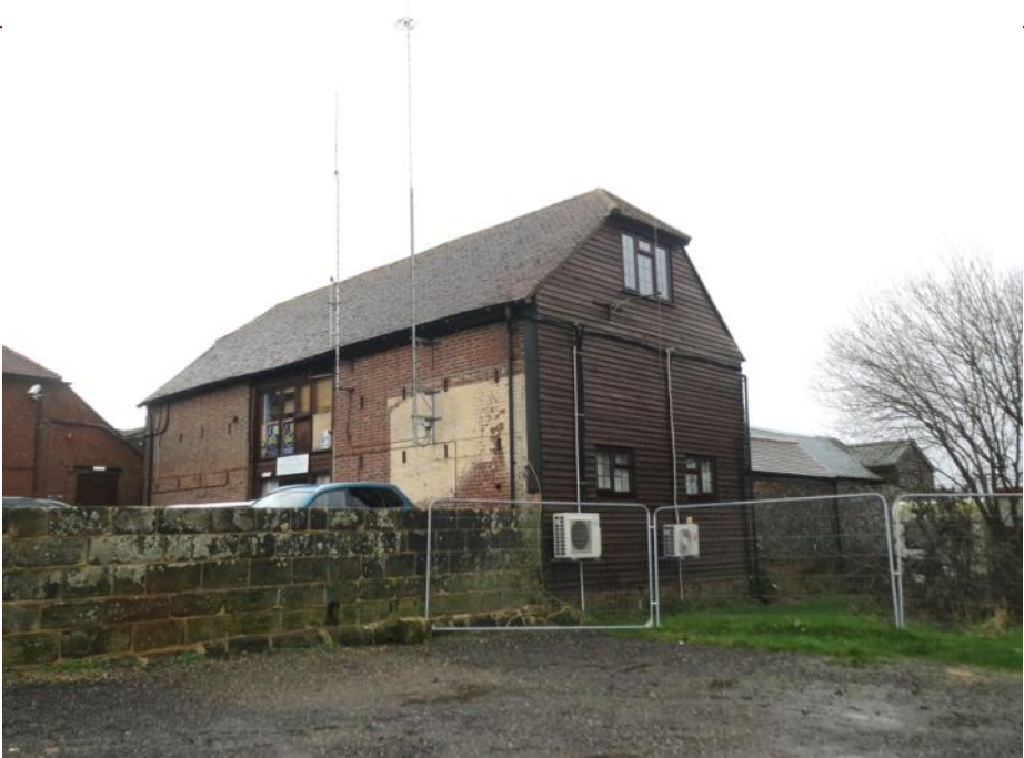
Figure 27: The barn at Bird in Eye Farm, seen from the north west
