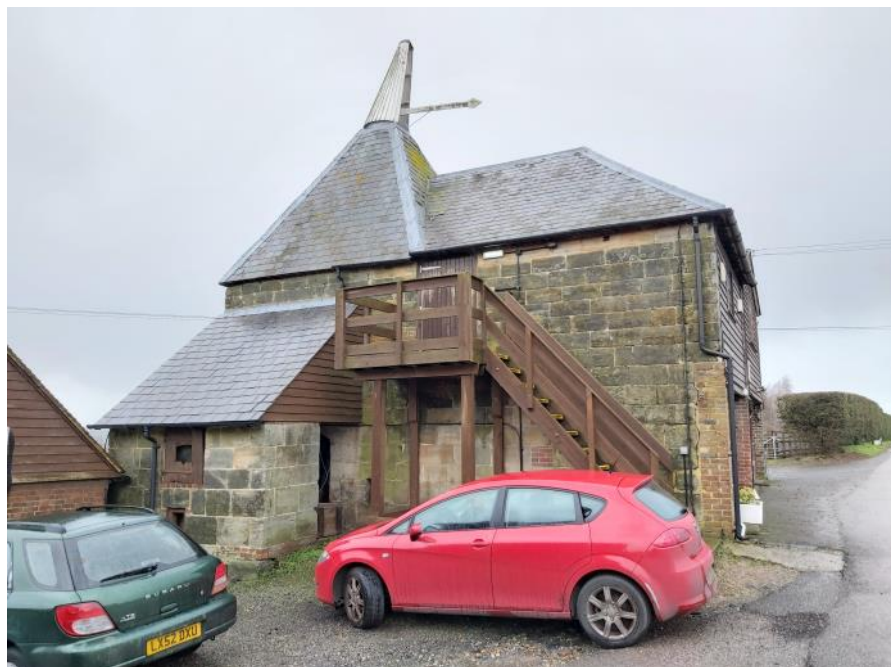
Figure 17: The south elevation of The Oast. The staircase is a modern replacement of one that would have been constructed in this location to provide access to the drying floor and the stowage area
