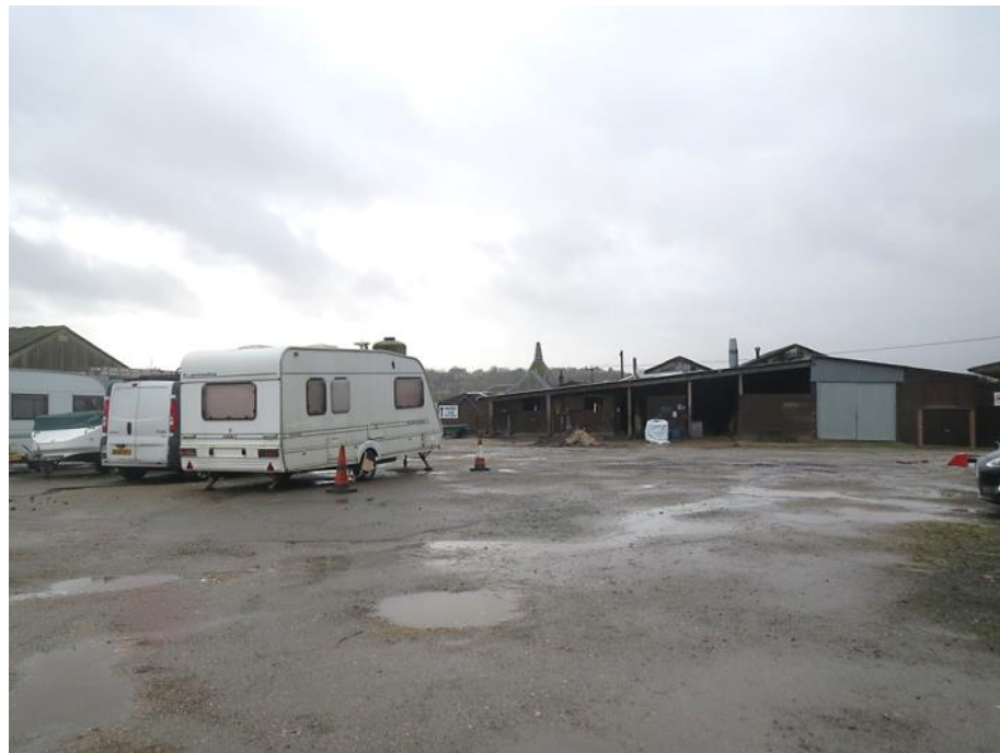
Figure 10: View into the yard to the east of the main section of the farmstead, seen from the track that runs alongside the eastern side of the farmstead, looking west. The upper section of the oast and the cowl can be seen from this point, within the context of the wider, diversified farm yard
