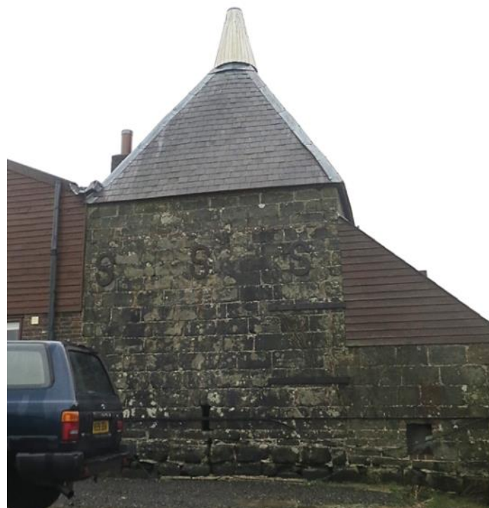
Figure 20: The west elevation provides the best view of the squared, coursed ragstone used in the construction of The Oast
