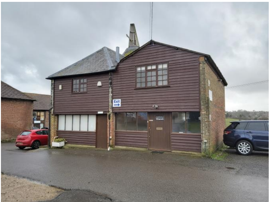
Figure 18: The east elevation of The Oast. The right hand half of the building was a later addition to the original structure
