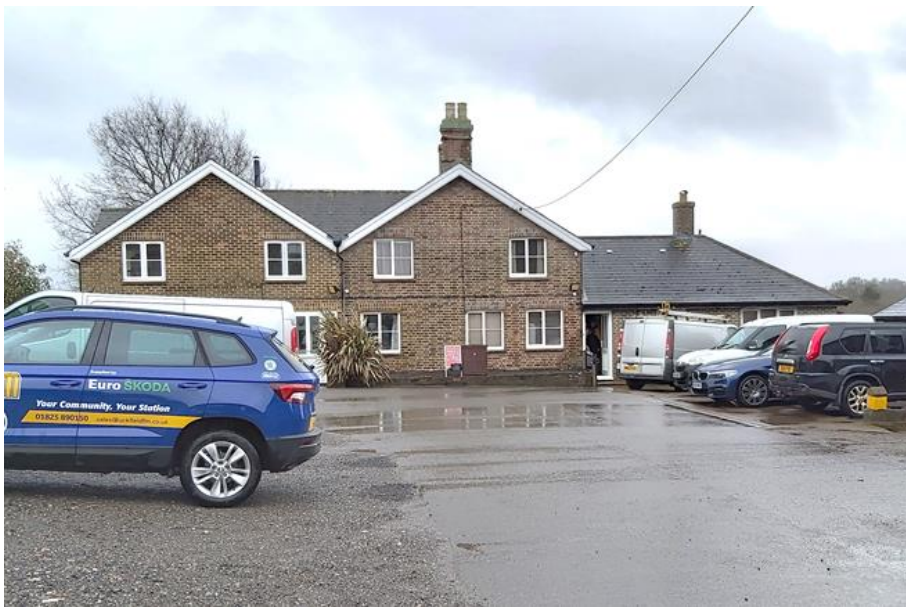
Figure 8: North elevation of Bird in Eye Farmhouse
