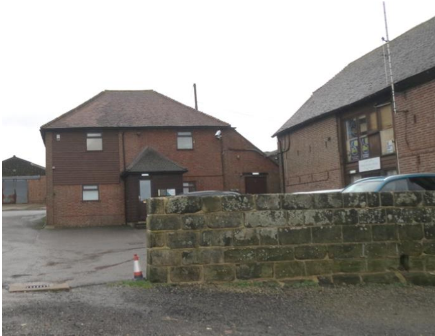
Figure 23: There is a stretch of walling constructed from squared, coursed ragstone to the south of The Oast, that runs along part of the edge of the original farmstead
