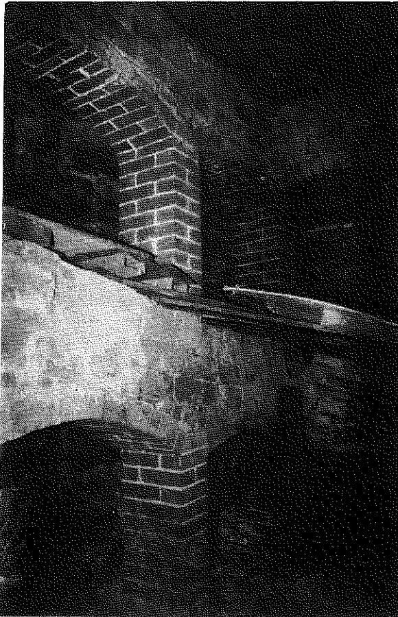
10iii: The rise of the flues on the west side of the kiln.
