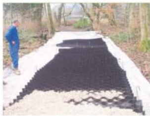
CellWeb during installation.
