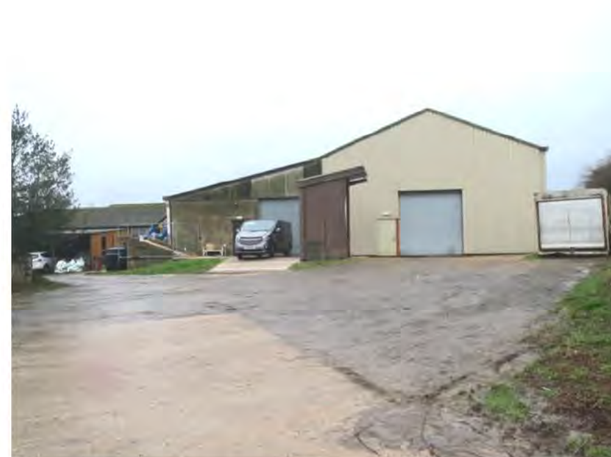
Figure 6: One of the large span modern farm buildings at Bird in Eye Farm, seen from the south
