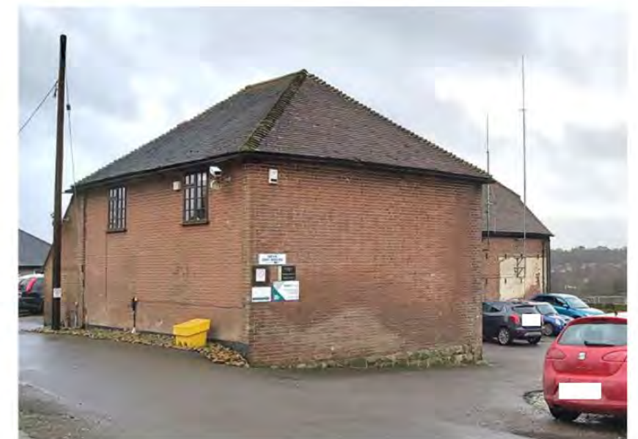
Figure 26: The former farmhouse within the centre of the farmyard. The brick building sits on a plinth of squared, coursed ragstone
