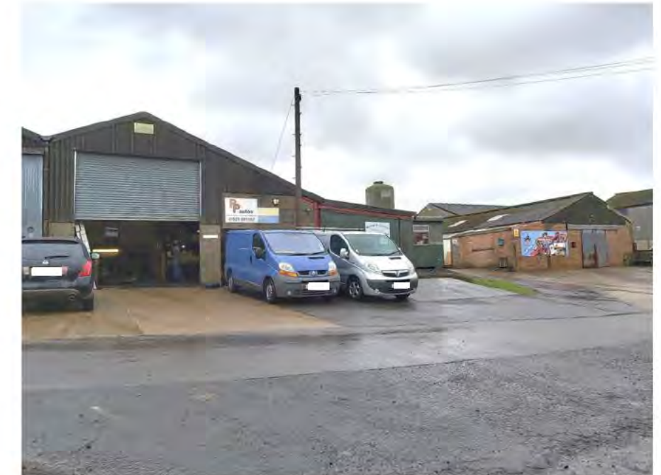
Figure 7: Large span modern farm buildings at Bird in Eye Farm, immediately opposite The Oast, seen from the west
