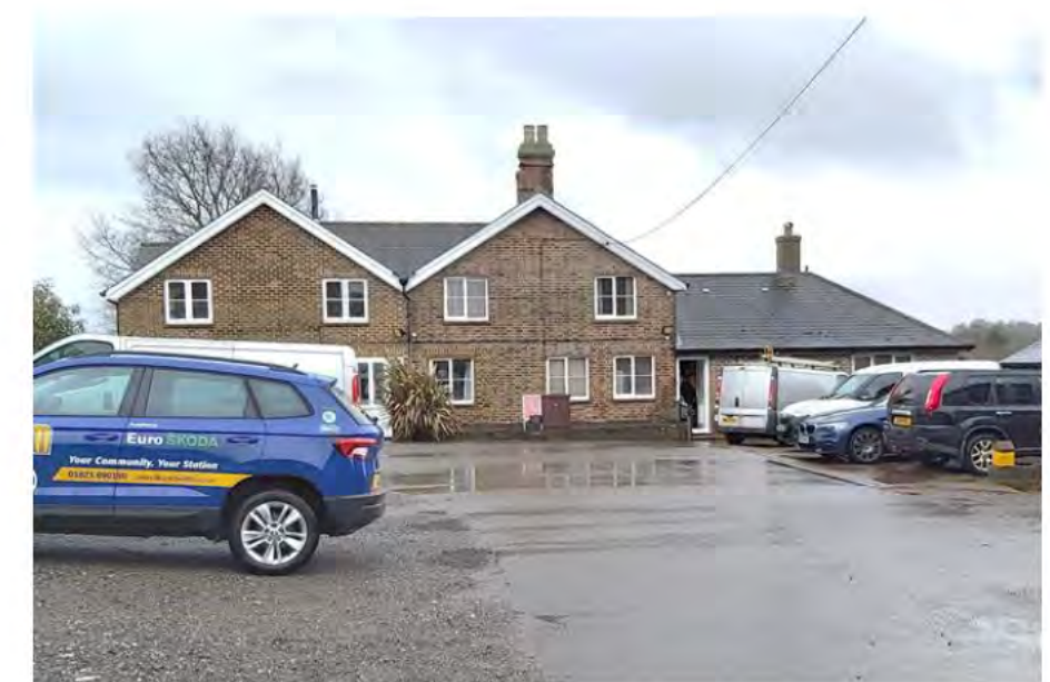
Figure 8: North elevation of Bird in Eye Farmhouse
