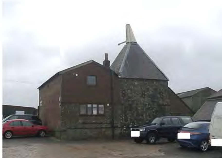
Figure 16: The west elevation of The Oast
