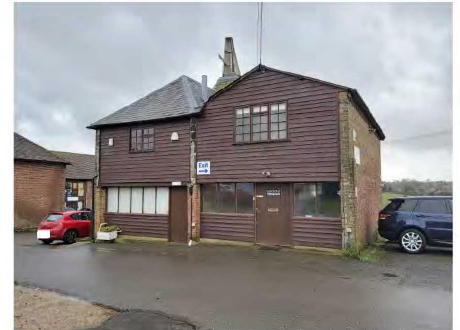
Figure 18: The east elevation of The Oast. The right hand half of the building was a later addition to the original structure
