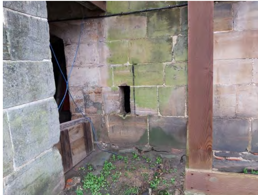
Figure 20: The entrance into the kiln via the lean to on the south side of The Oast. This would have been a blank opening originally, with no doors which lead into a lobby which was shielded from the furnace by two metal doors
