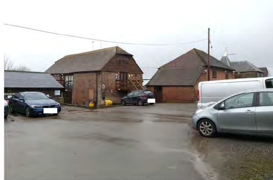
Figure 28: The barn seen from the south east, adjacent the former farmhouse
