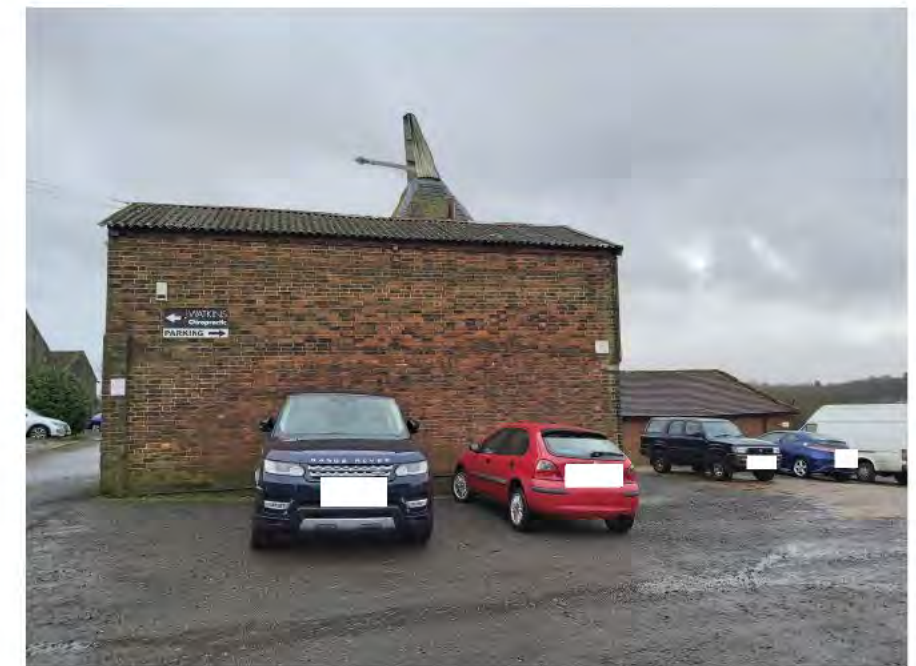
Figure 19: North elevation of The Oast
