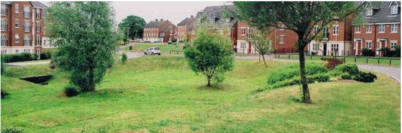
Detention Basin (image courtesy of Morton-Roberts Consulting Engineers Ltd)
