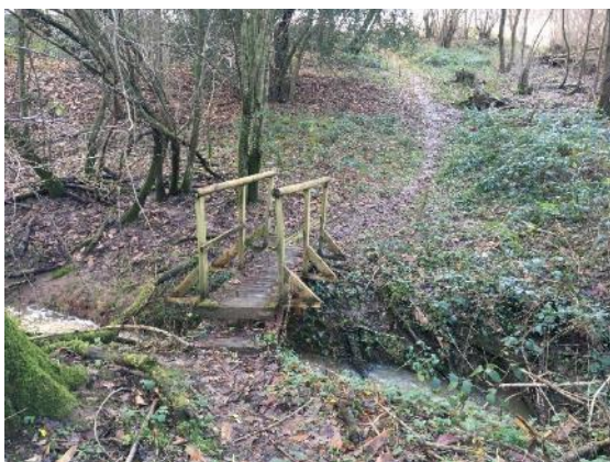
Photograph 7. Existing footbridge over stream, along footpath through Ancient Woodland W2.
