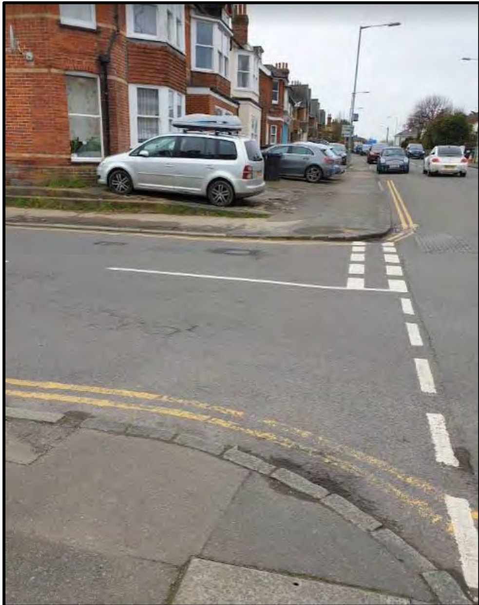
Figure 7: Existing Pedestrian Crossing at Harcourt Road
