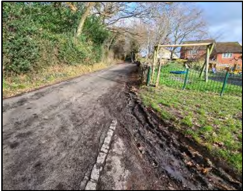
Figure 22: Hempstead Road at Access to Play Area
