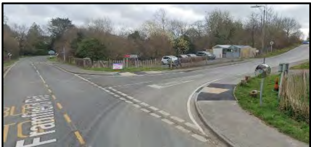
Figure 5: Existing Pedestrian Crossing at Access to Uckfield Hospital
