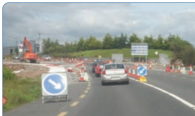
Road works in Ireland
