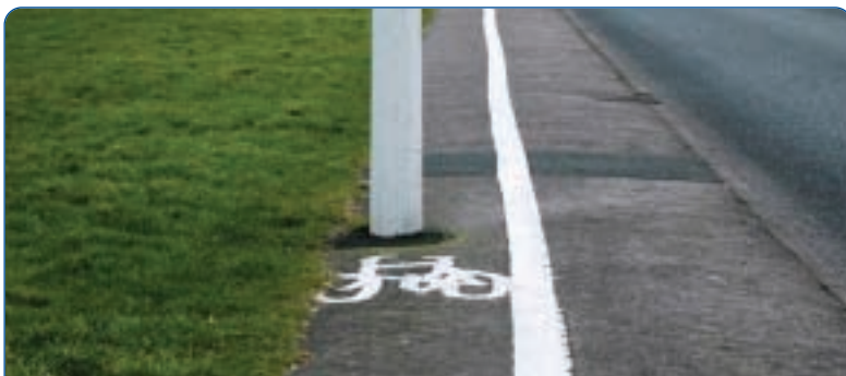
Poor quality cycle facilities
