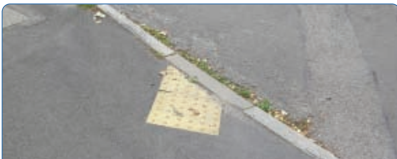
Minimalist approach to tactile paving
