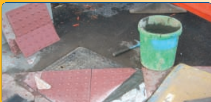
Cutting tactile paving to fit a chamber cover following a design stage Road Safety Audit that expressed concern for blind pedestrians stepping into the carriageway without realising
