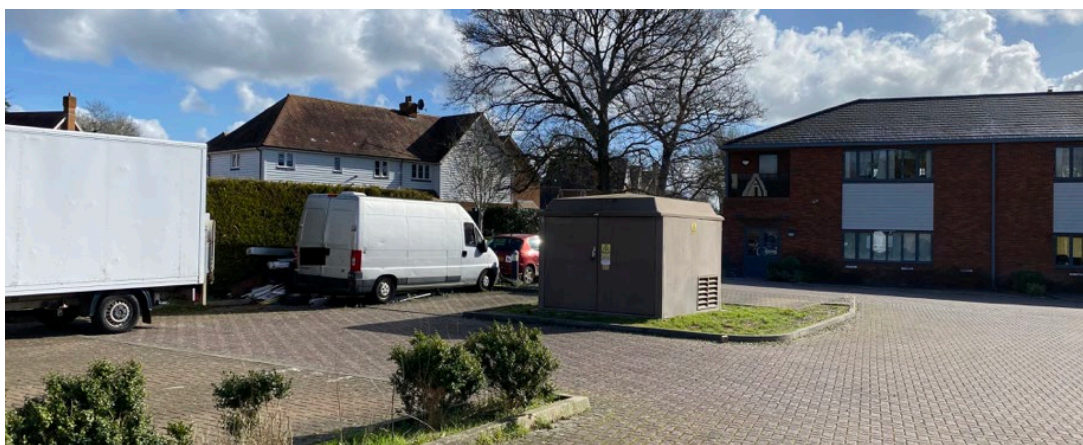
Carriers Way electrical substation
