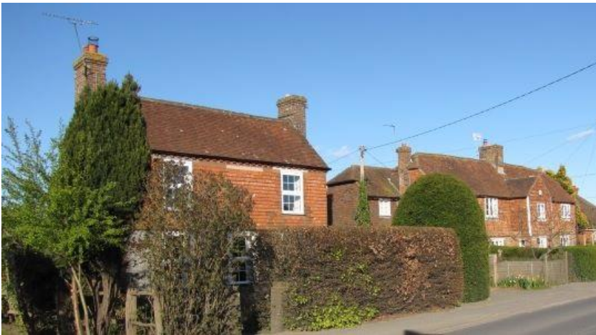
Early c19th house and row of three c18th cottages with tile-hung first floor, brick groundfloor and clay tiled roofs, some gabled, some barn-hipped. Mainly hedging on front boundary with kerbed pavement
