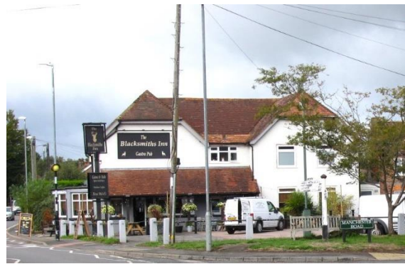
1930s public house with barn-hip roofs
