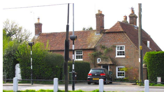
C17th and c18th brick dwellings with clay-tiled roofs (left is a single house, right 3 cottages) with mixture of gables and barn-hips, one behind garden wall and the other a hedge
