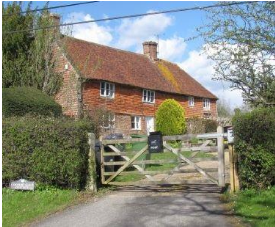
Examples of c18th cottages with clay tile-hanging on first floor behind mixture of hedges and rustic timber fencing
