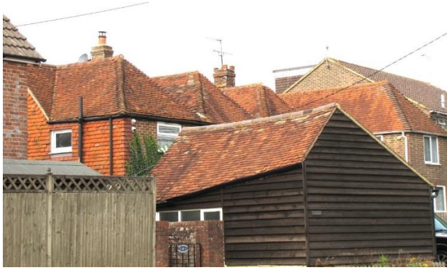
These cottages have a distinctive series of hipped roof projections which is found on a number of old cottages in Ninfield, sometimes with gables
