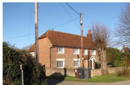
Early c19th brick farmhouse and converted barn with typical 'barn-hip' clay-tiled roofs behind front boundary wall and hedge on back road without kerbs
