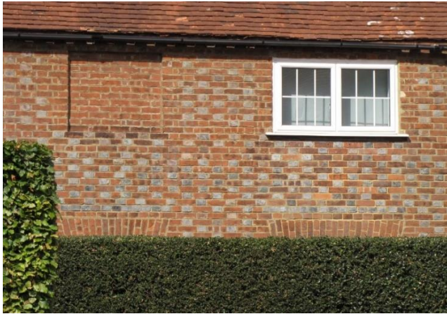
Left photo - Early-mid c19th brickwork with grey brick headers (in numerous variations of Sussex Bond) is typical of many local buildings of this period. Right - late c19th brickwork
