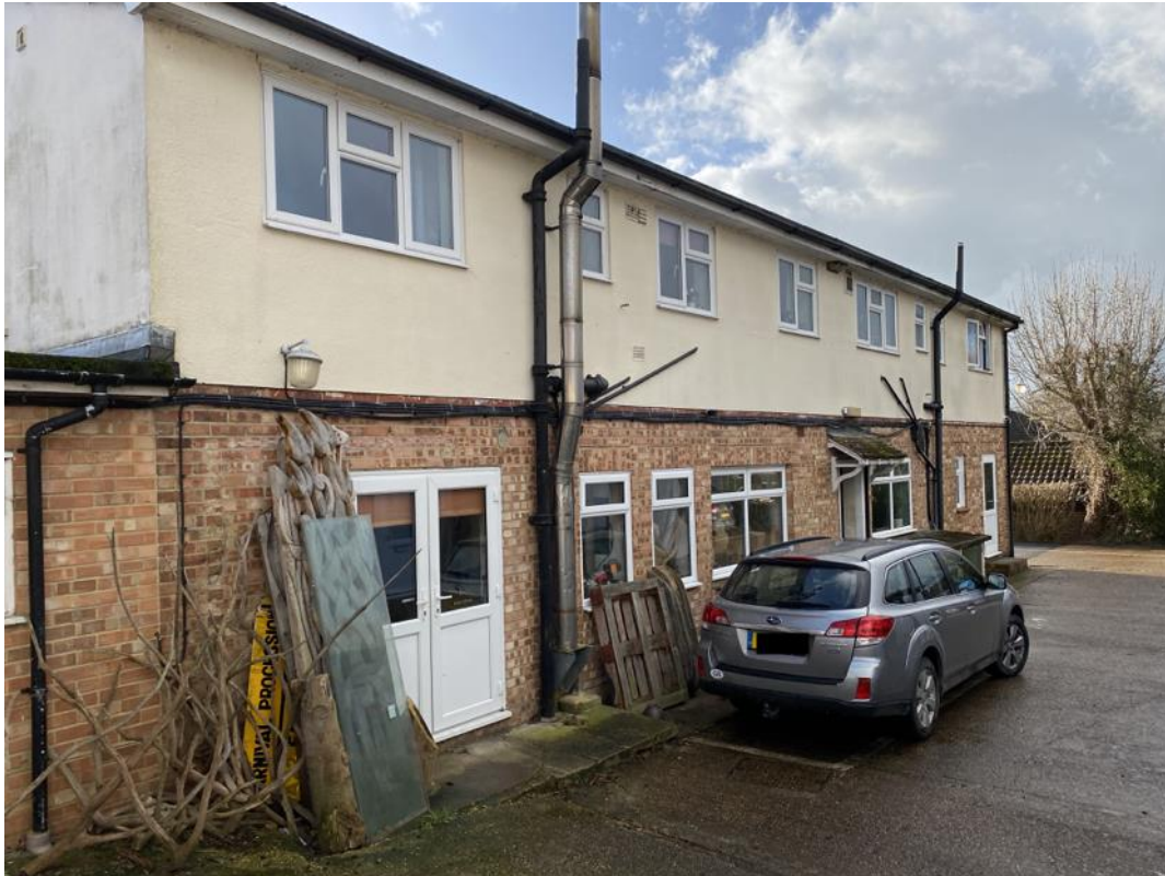
Rear of Village Works
