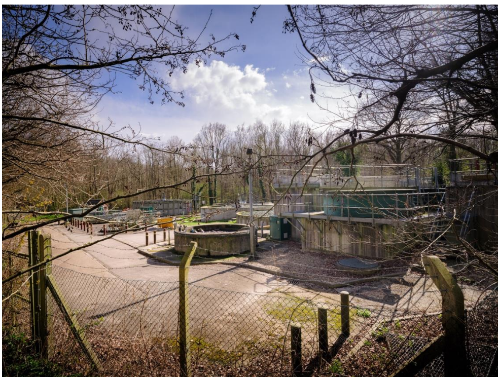
East Hoathly Sewage Treatment Plant
