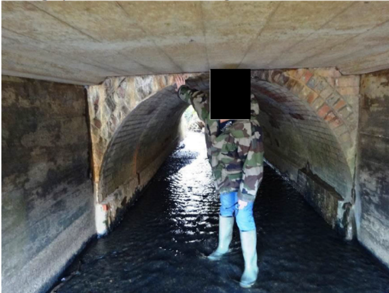
Photograph 5 - Stream Farm Bridge
