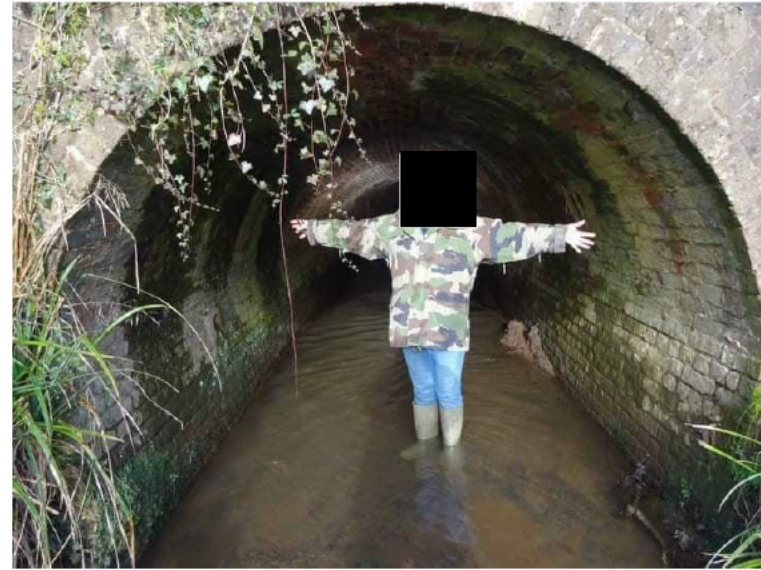
Photograph 6 - Culvert under Cuckoo Trail
