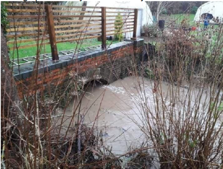
Photograph 7 Railway culvert in heavy rain conditions
