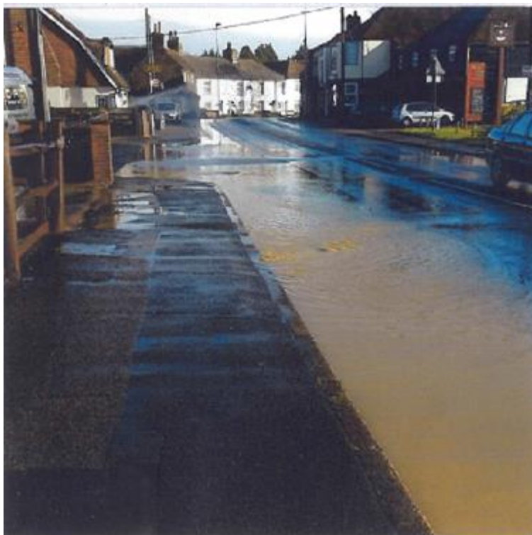
Feb 2012 – View looking East along A271. Failure of highway drains due to river high level. Photograph provided by resident of Lower Horsebridge.
