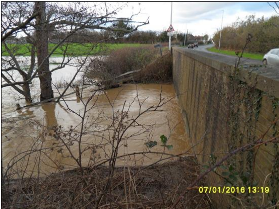
Jan 2016 – Water level downstream of A271 crossing. Photograph provided by S Carr.
