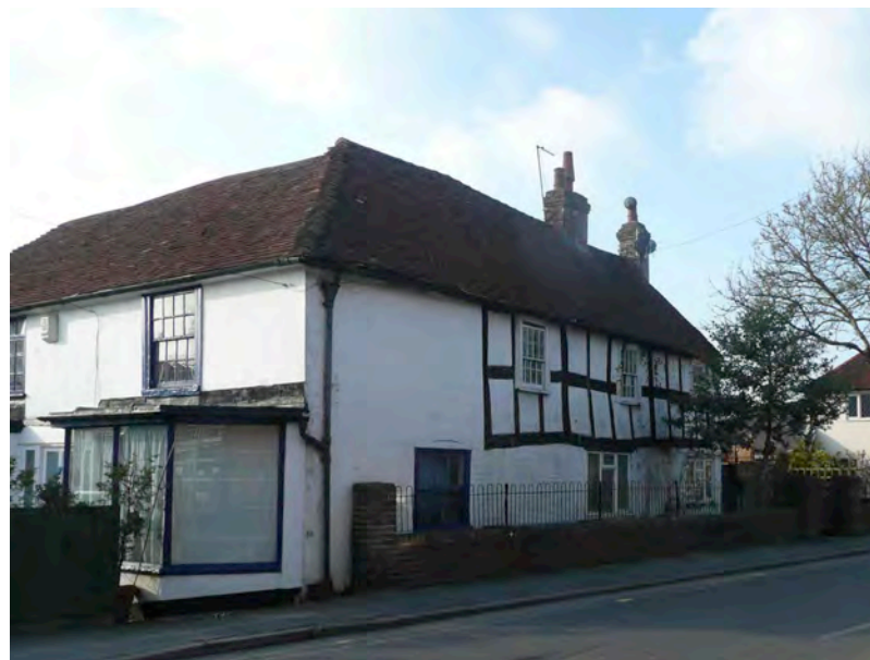
Fig 45: The Spa Stores dating from circa. 17 th century with its exposed timber box framing to one side.
