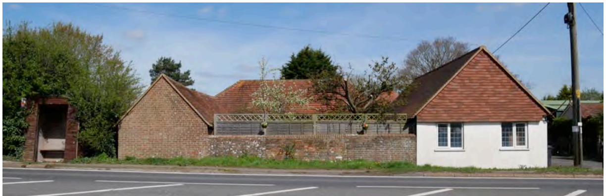
Fig 29. Former farm buildings of a U-shaped plan form with access to the Common.
