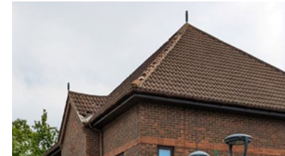
Hipped roof with concrete tiles
