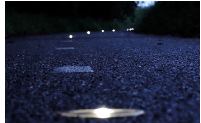
Figure 132: Example of a foot/cycle path which is lit by solar cat's-eye providing some light for pedestrian and cyclists without creating any disturbance to the nearby properties or unacceptable levels of light pollution.
