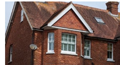
Sash windows with wooden detailing
