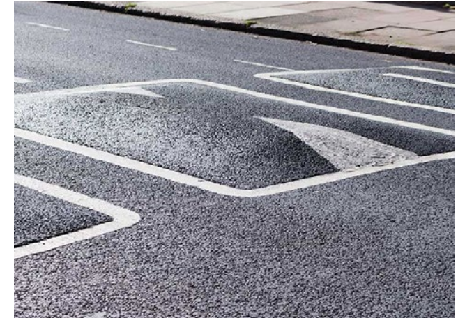
Figure 59: Example of a speed cushion.
