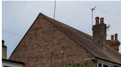
Gabled roof with brown clay tiles
