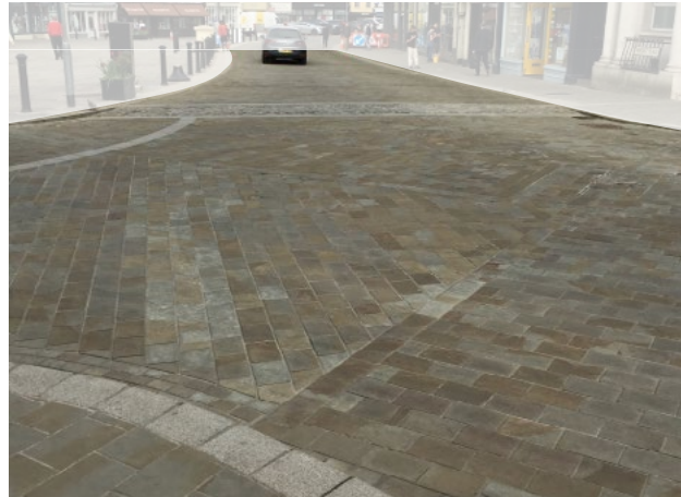
Figure 57: Example of a junction improvement with raised pedestrian crossing and use of different styles of stones to create markings and facilitate movement, elsewhere in UK.
