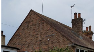
Gabled roof with brown clay tiles
