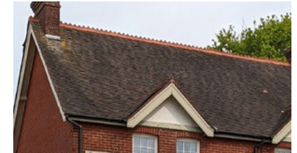
Gabled roof with dark slates
