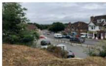
4. A view of the High Street from the main A267 through the village, showing the fairly tight-knit frontage buildings with commercial ground floor uses
