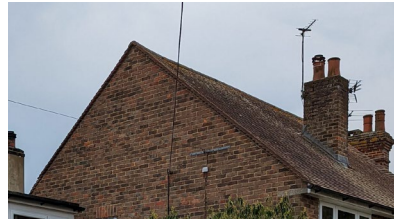
Gabled roof with brown clay tiles
