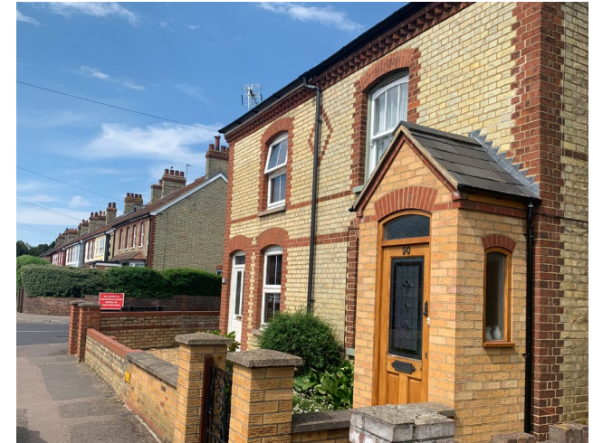
Figure 116: Positive example of a front extension.
