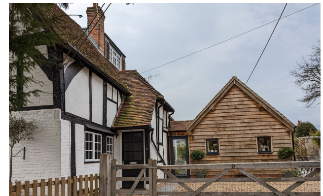
Figure 118: Positive example of a side extension that respects the existing building in terms of scale and building materials.
