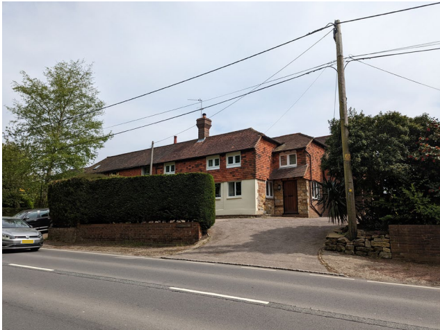
Figure 123: Local example of low height red brick wall and hedgerow boundary treatment.
