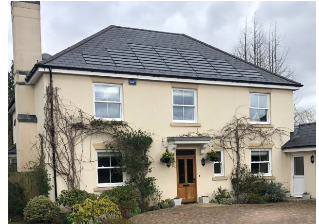
Figure 138: Use of shingle-like solar panels on a slate roof, with the design and colour of the solar panels matching those of the adjacent slate tiles.
