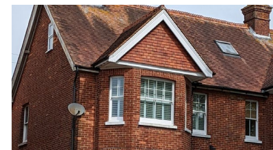
Sash windows with wooden detailing
