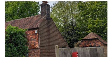
Catslide roof (main property) and dutch roof (out-building)
