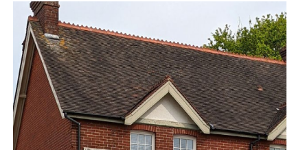
Gabled roof with dark slates
