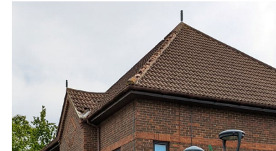
Hipped roof with concrete tiles
