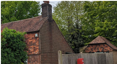
Catslide roof (main property) and dutch roof (out-building)
