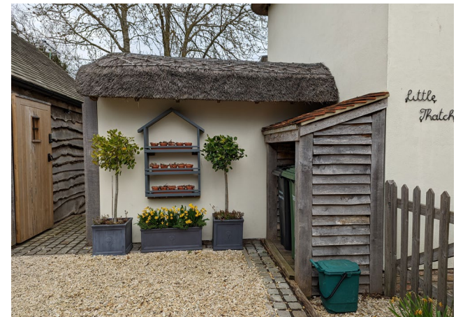
Figure 79: Example where the bins are stored under the shed, whilst the side wall is decorated with flowers and plants to improve the environment. This arrangement combined with the particular permeable paving contributes a rural feel.
