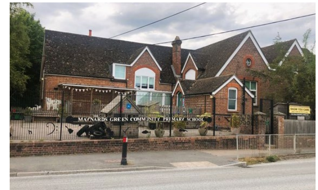
Figure 26: Maynard's Green Primary School.
