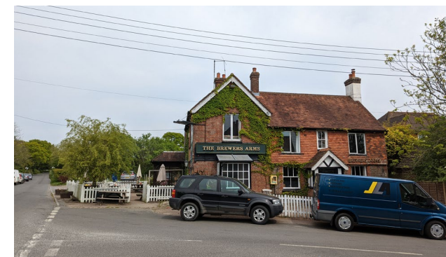
Figure 30: View to Brewers Arms Public House which is located to the junction of Nettlesworth Lane and Foords Lane acting as a landmark building and a focal point for the village.
