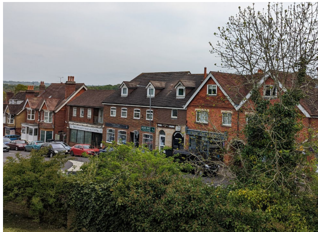
Figure 23: Local example of a continuous roofline which often gets interrupted with chimneys, dormers and pitches.
