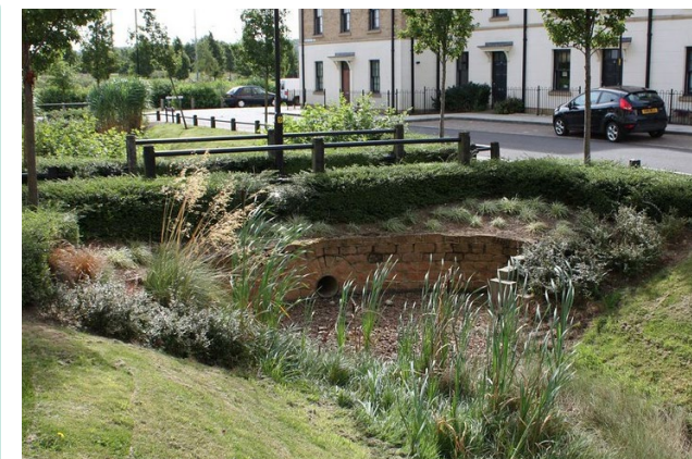
Figure 84: Example of swales check dam integrated with a crossing point, somewhere in UK.
