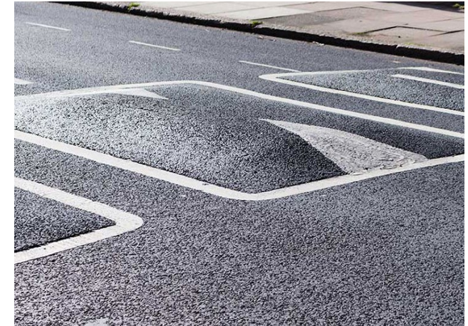
Figure 59: Example of a speed cushion.
