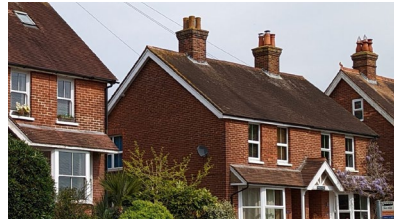
Gabled roof with red clay tiles
