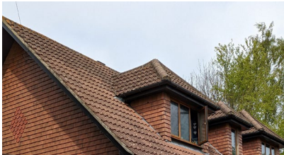
Gabled roof with red clay tiles and hipped dormers
