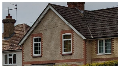
Yellow brick with red brick dressing around windows
