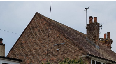
Gabled roof with brown clay tiles
