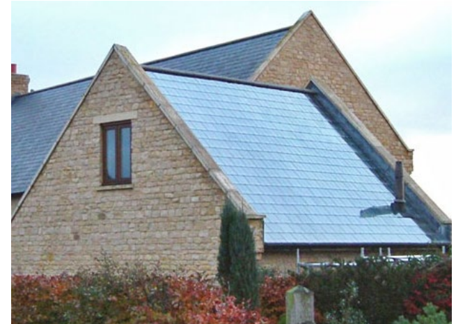
Figure 139: Positive example of implementing solar panels since the design stage.
