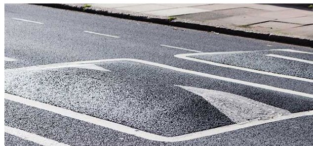
Figure 143: Example of speed cushion.
