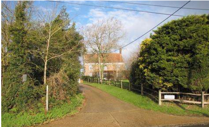
Luxford House (former Lower Standard Hill Farmhouse) Grade II* from A269
