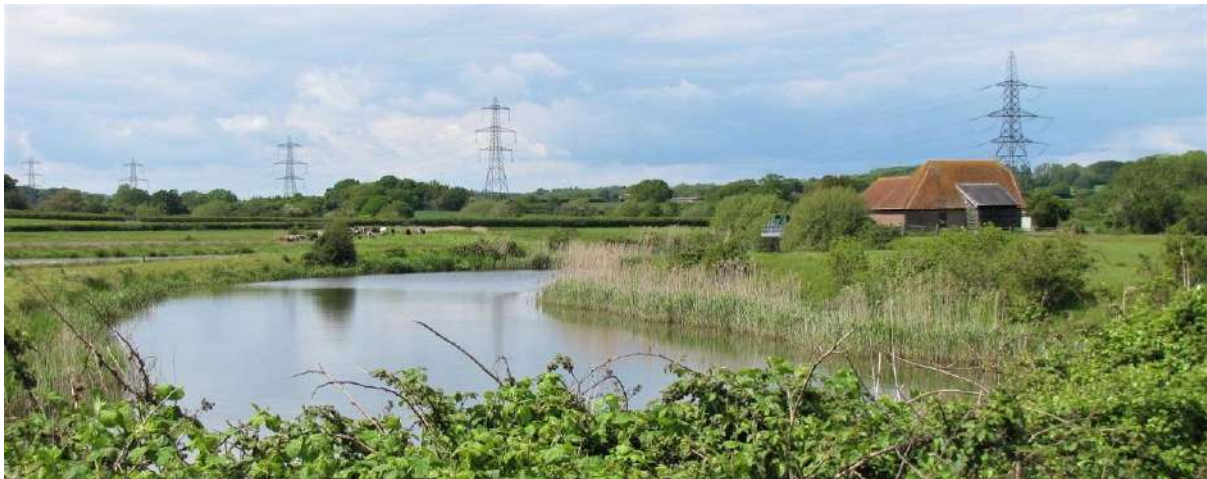
Waller's Haven river and Pumping station looking north towards A271 and AONB
