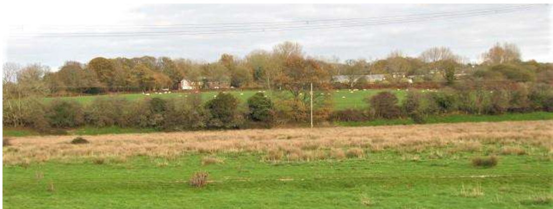
Hazards Green Waterworks viewed from Wallers Haven levels to SW
