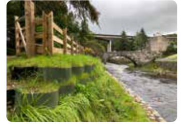
Webwall Retaining Walls
