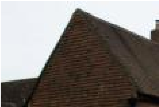
Plain mortared verge without barge boards
