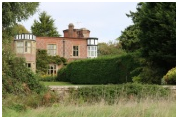
Ha-ha wall to the garden of Parkfield and Brent House
