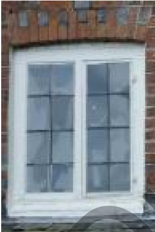
Window - pegged frame with side hung casements with square quarries of glass within lead comes
