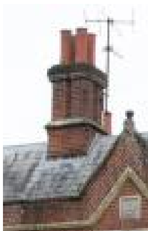
Decorative brick chimney stack with clay pots
