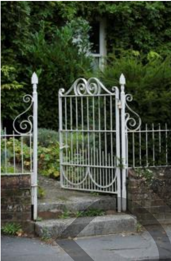
Gate and railings at Sandrock
