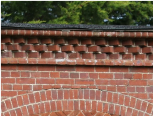
Brick dentilation course
