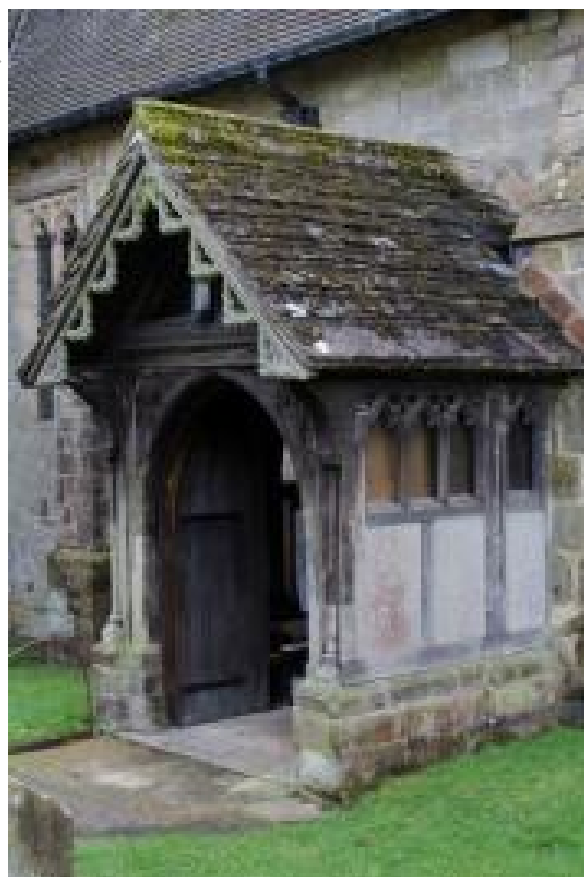
Horsham stone slate on church porch
