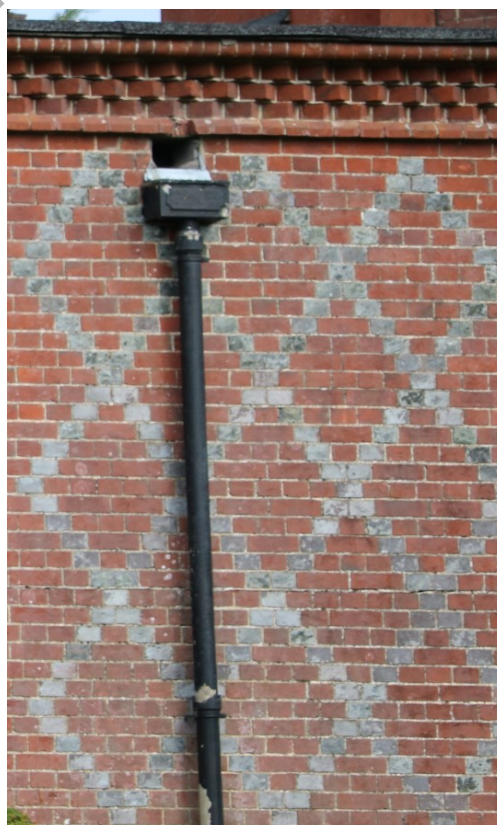
Diaper brickwork
