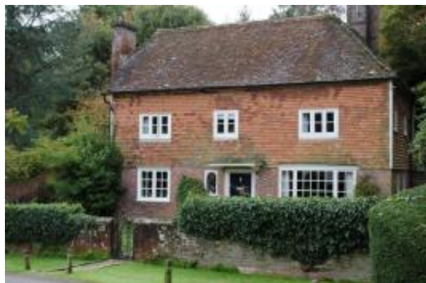
Boundary wall at Forge Cottage
