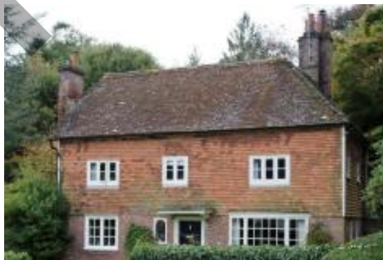
Chimneys and pots on a hipped roof
