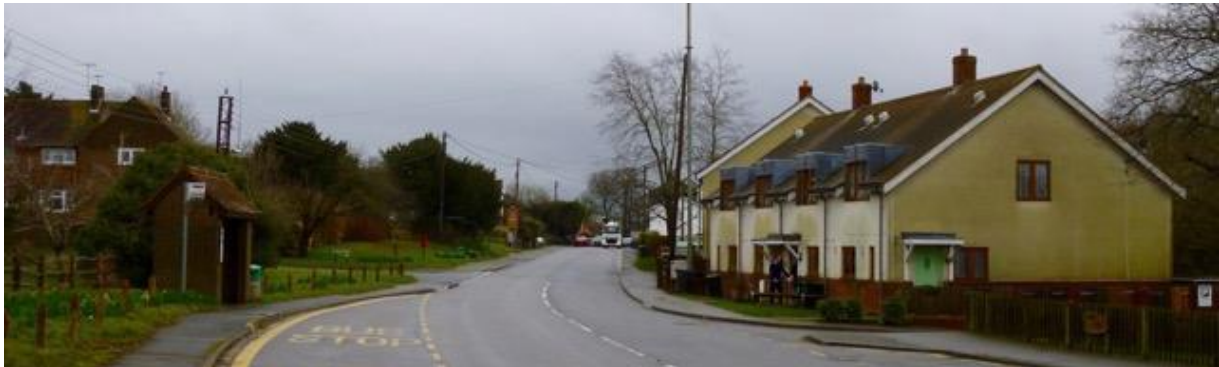
North Lodge, Hailsham Road, Herstmonceux.
