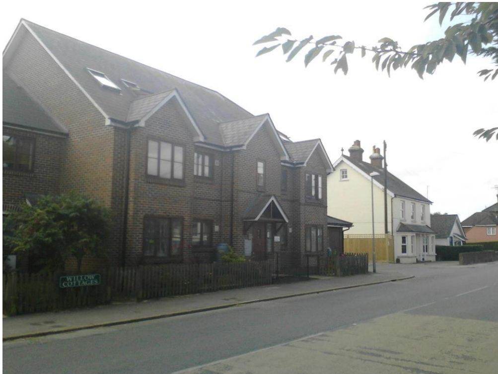
Second half of development on the road, showing flats and access road to bungalow development at the rear.
