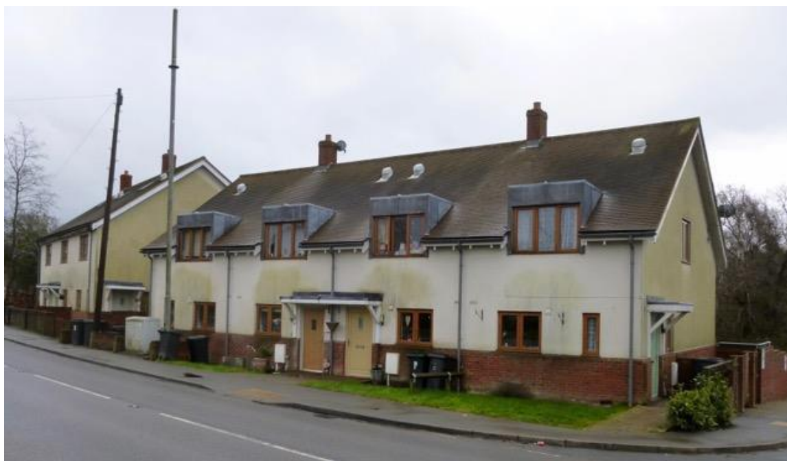
Inappropriate use of materials and design of dormer windows impacting on the outlook of North Lodge. Frontage of houses not finished off with suitable demarcation boundaries to pavement area.
