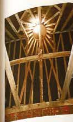
Fig 9.17 Great Dixter. Looking up the internal conical vent above the drying floor.
