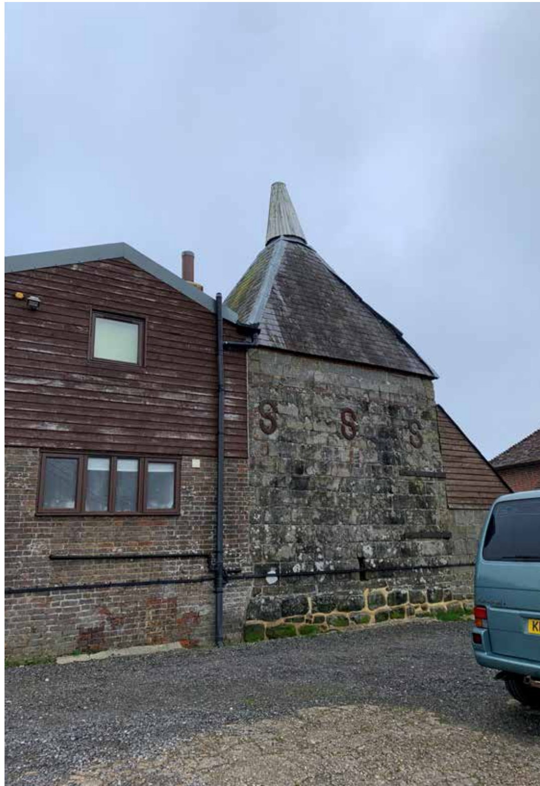
West elevation of the Oast House, Bird in Eye Hill
