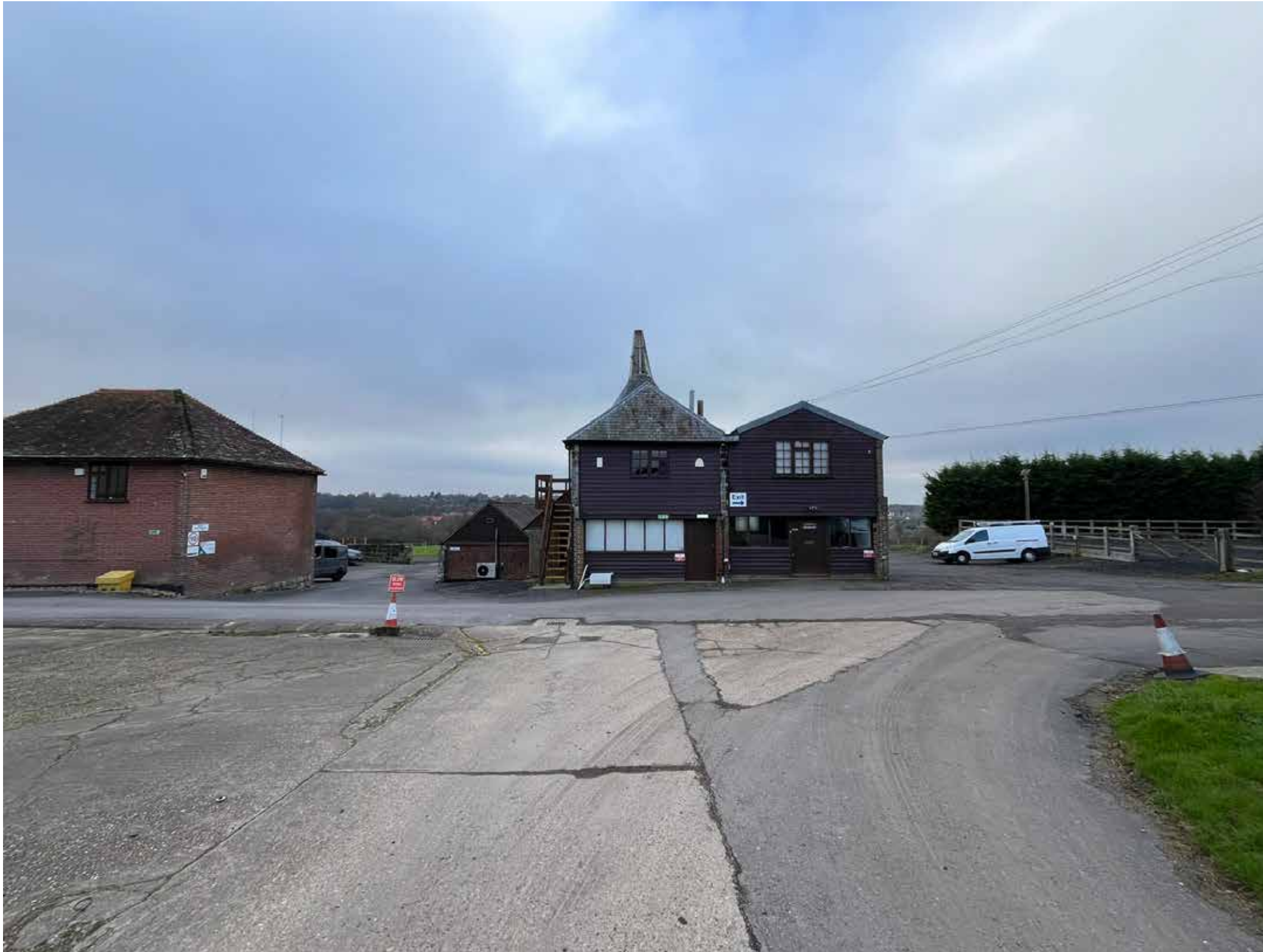
East elevation of the Oast House, Bird in Eye Hill and surrounding hard standing
