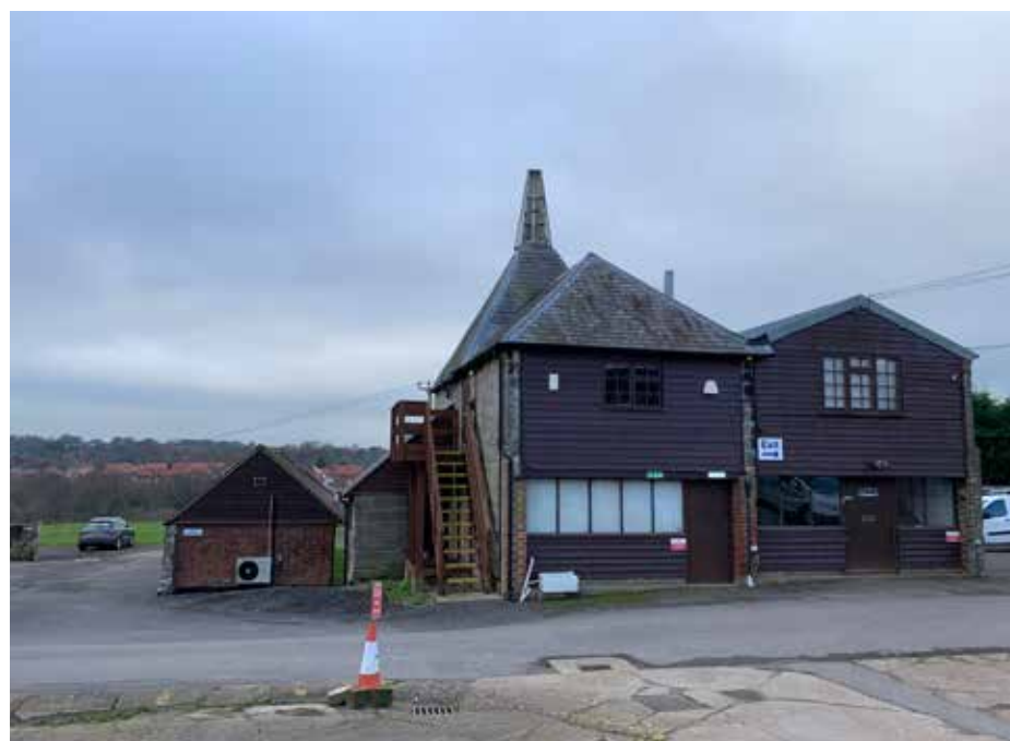
Figure 5.2 Northeast elevation of Oasthouse
