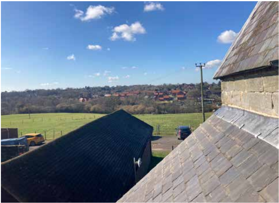
Figure 5.7 View from the Oast House external staircase
