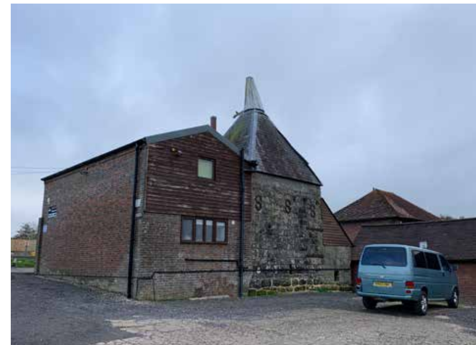
Figure 5.3 West elevation of Oasthouse
