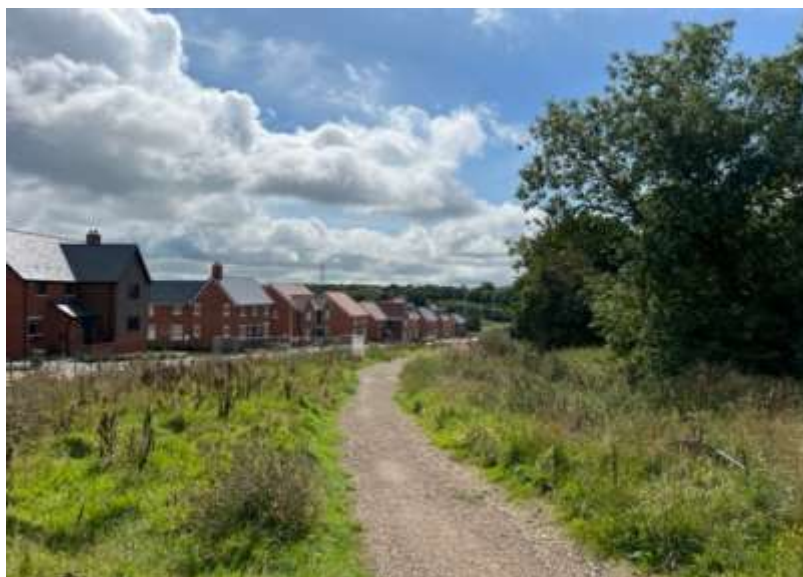
Figure 9. Development Fronting the AW, with footpath within the 15m buffer. No fencing to AW.
