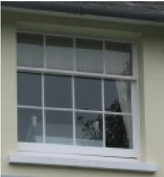
Multiple pane timber vertical sliding sash window
