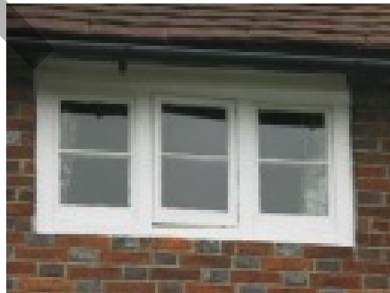
Simple side hung timber casement window with single central integral glazing bar
