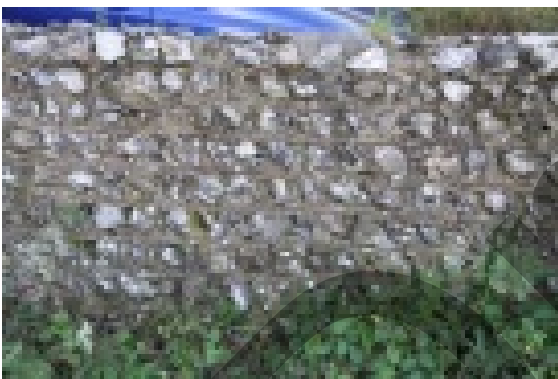
Flint boundary wall
