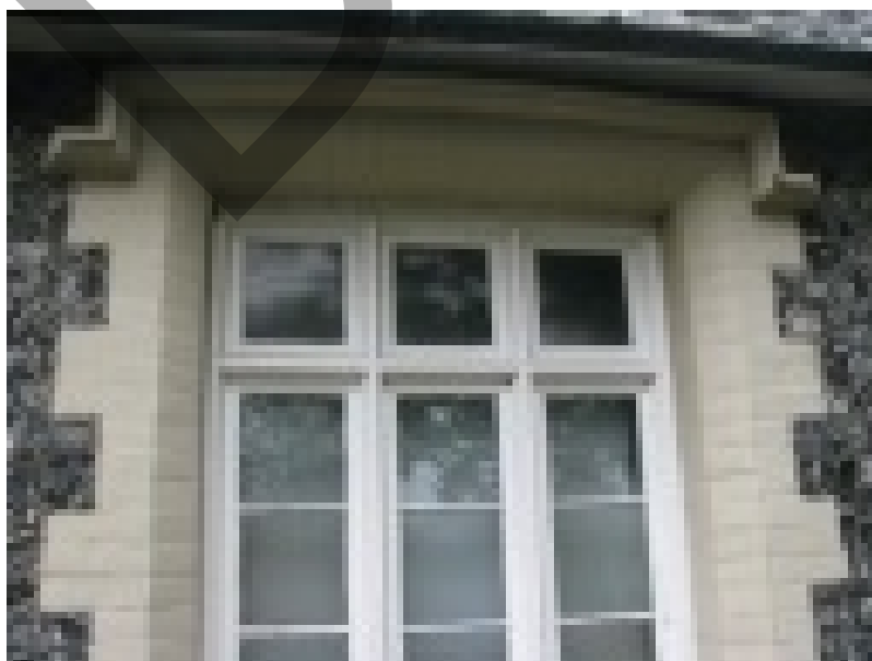
Timber mullioned window
