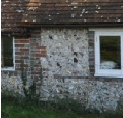
Flintwork with brick quoins
