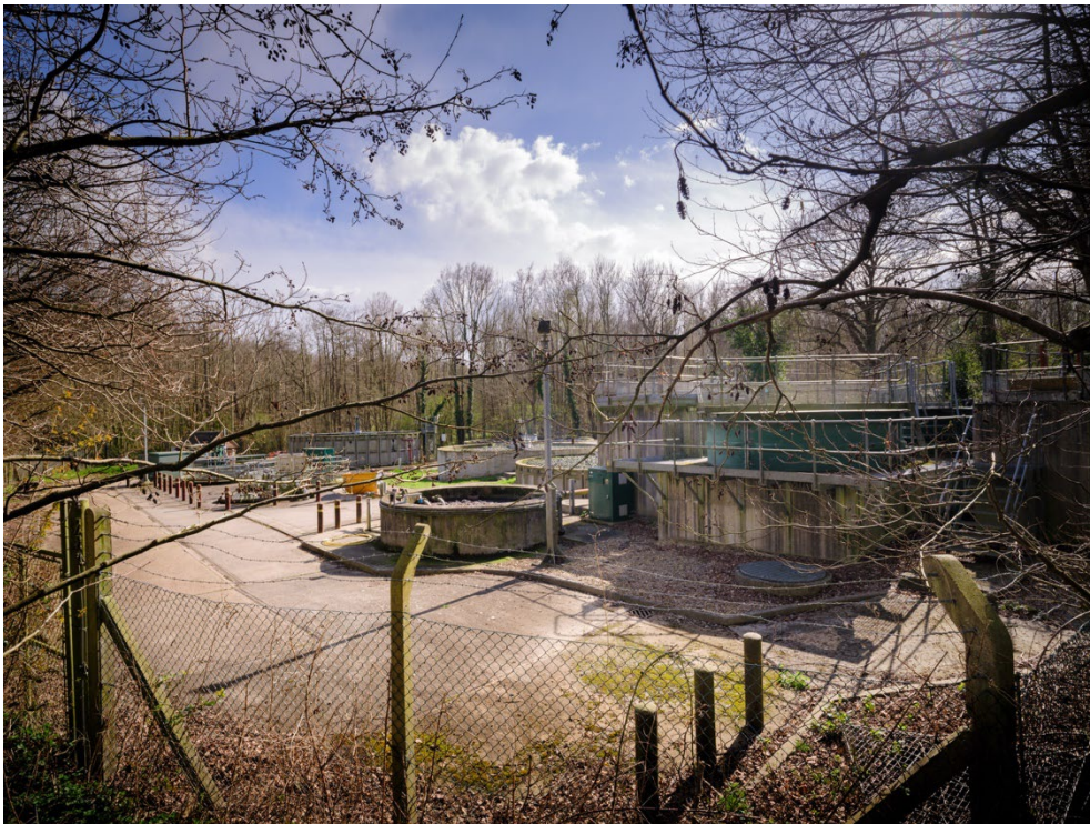
East Hoathly Sewage Treatment Plant
