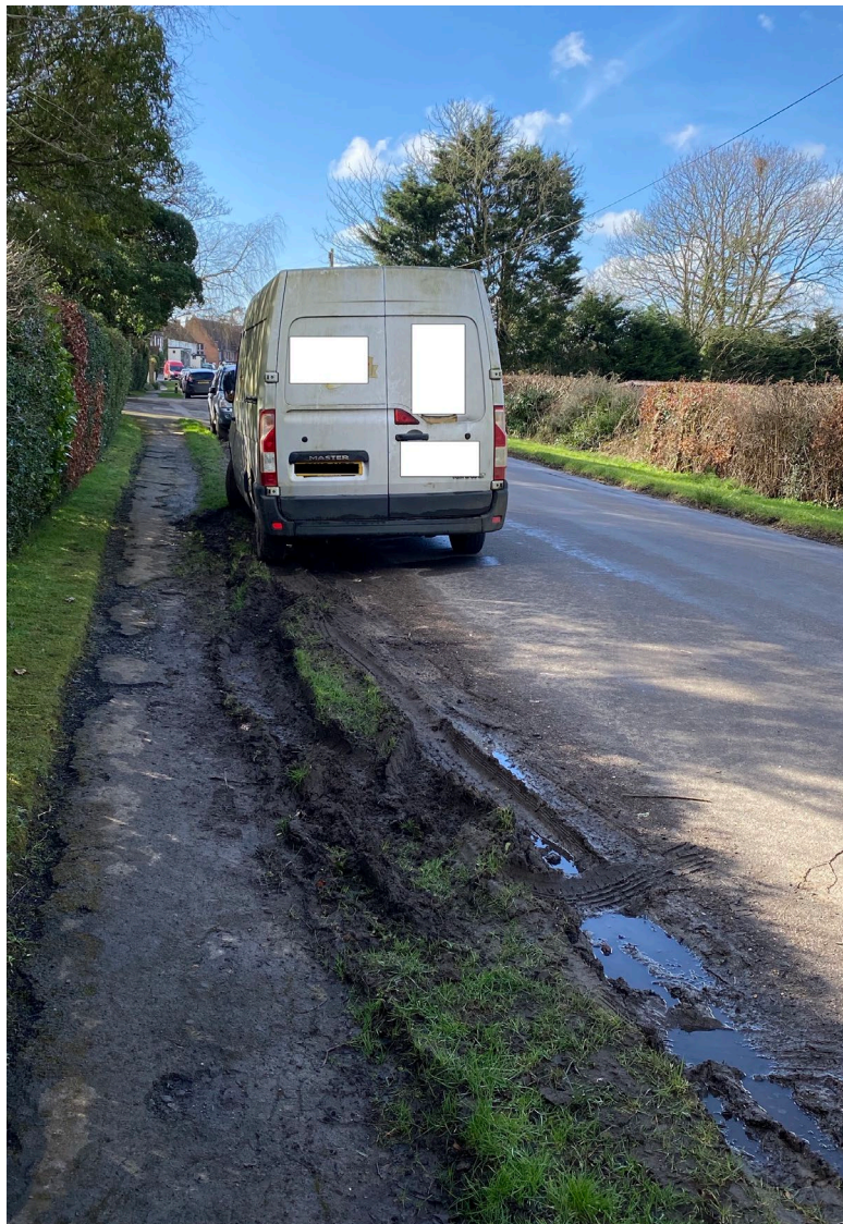
Damage to Verges on Waldron Road
