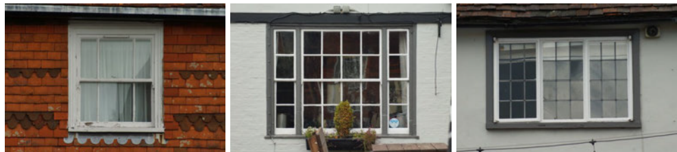
Double-hung sash windows
