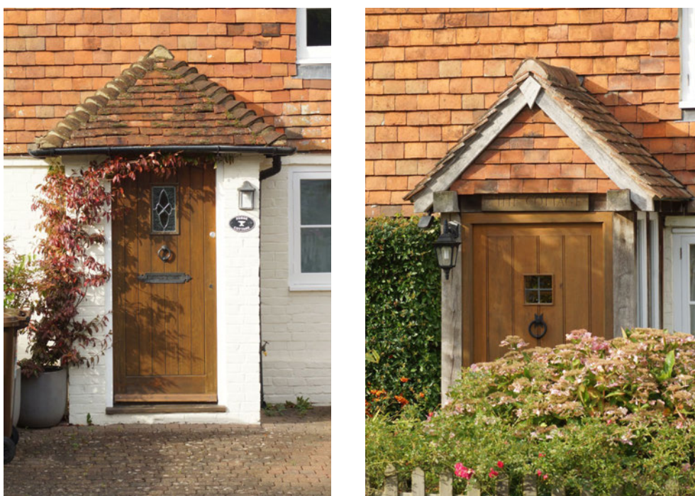
Traditional, enclosed porches with hipped roof (l) and gable ended roof (r).
