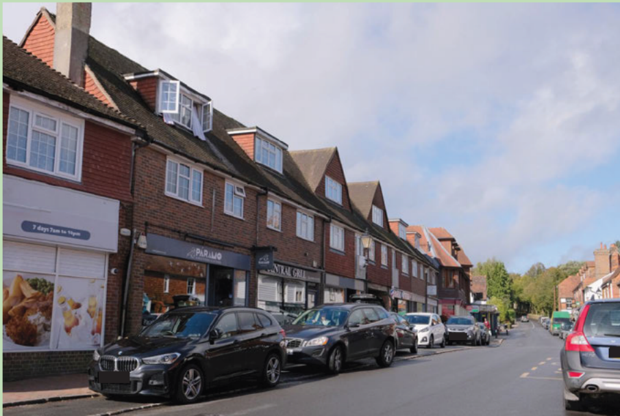
1950s development on the south side
