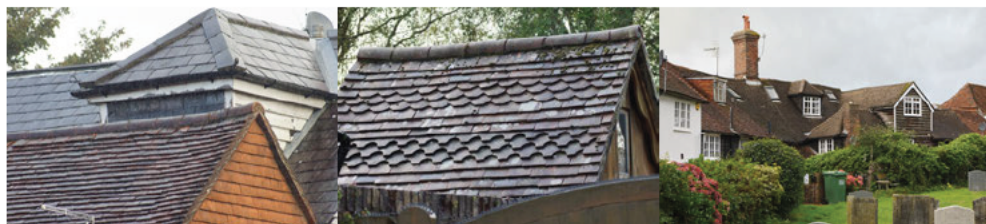
Roofs of Wadhurst, primarily red clay tile with grey slate as a secondary material.
