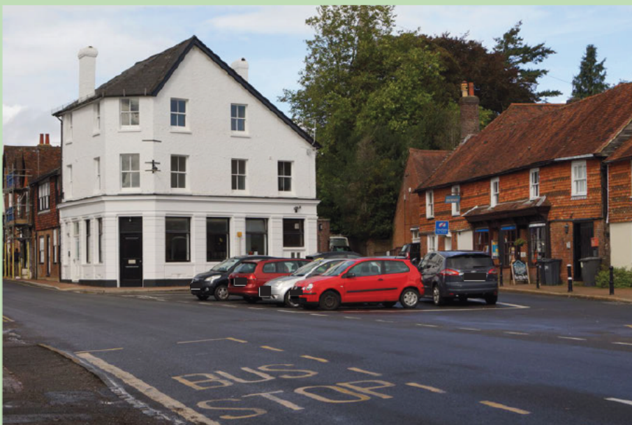
Parking in the town square, view looking north west
