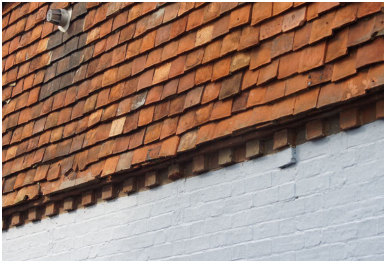
Brick headers used to form a dentilled course below the hung tiles.
