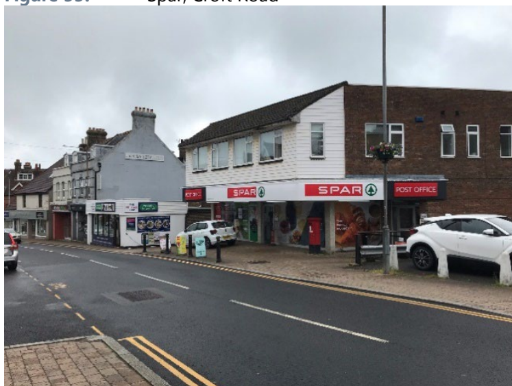
Figure 55. Spar, Croft Road
