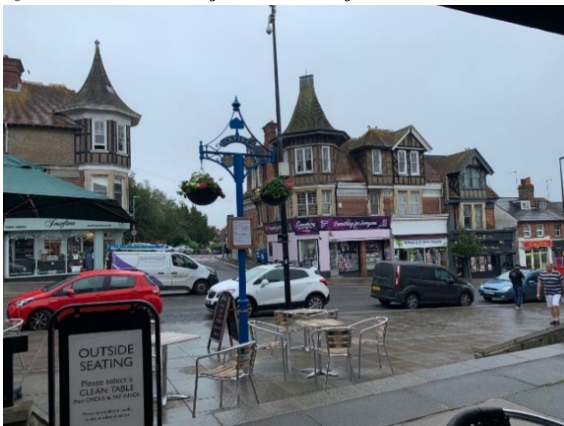
Figure 43. View east from High Street towards Grange Road
