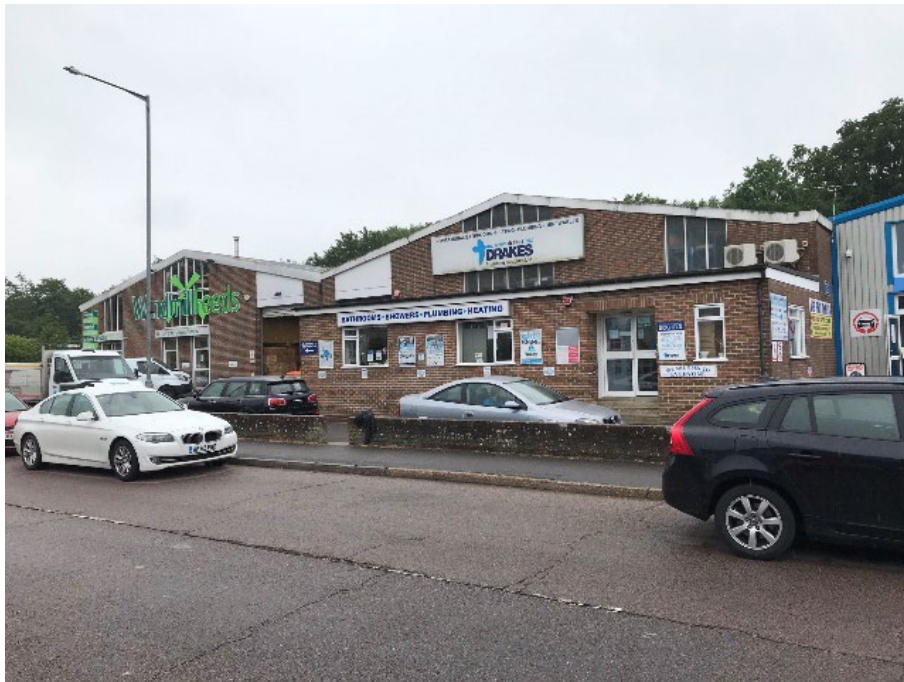
Figure 44. Retail units in the Bellbrook Retail Park
